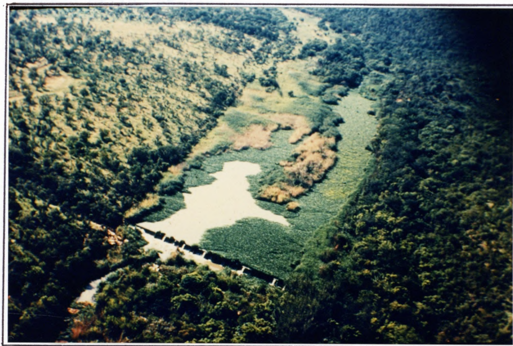
d. Thornhill Dam, Hectorspruit 17-12-1985
