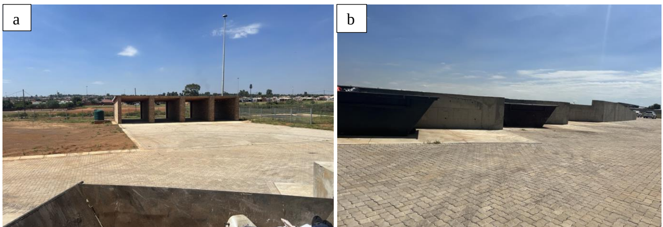
Figure 4.16a) Waste sorting station for the Mhluzi Waste Transfer Station b) Waste disposal section of the Mhluzi Waste Transfer Station.
