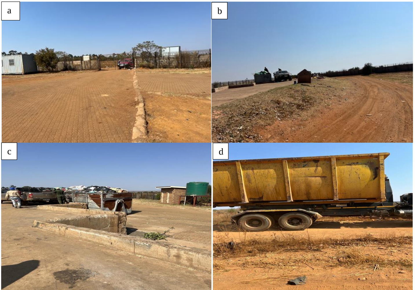
Figure 4.12a) Vehicle entering the Dennisig Waste Transfer Station to dispose of waste b) The pathway for the vehicles going to the platform c) Vehicles offloading the waste onto the large skips d) Waste collection done by the municipality.
