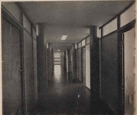
CORRIDOR FRIEZE LIGHTS IN PARTITIONS, PORTHOLES TO REDUCE GLARE
