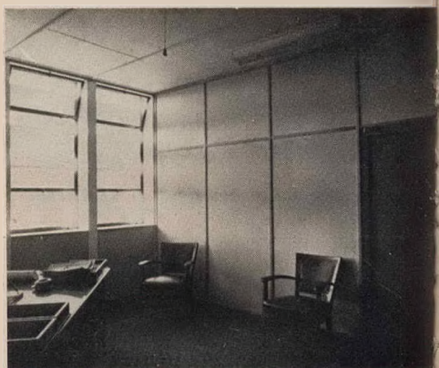
A TYPICAL OFFICE SHOWING MODULAR PARTITION AND WINDOW UNIT
