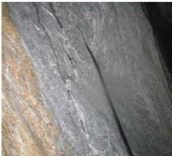
C) Phenomena of spalling in tunnel faces
