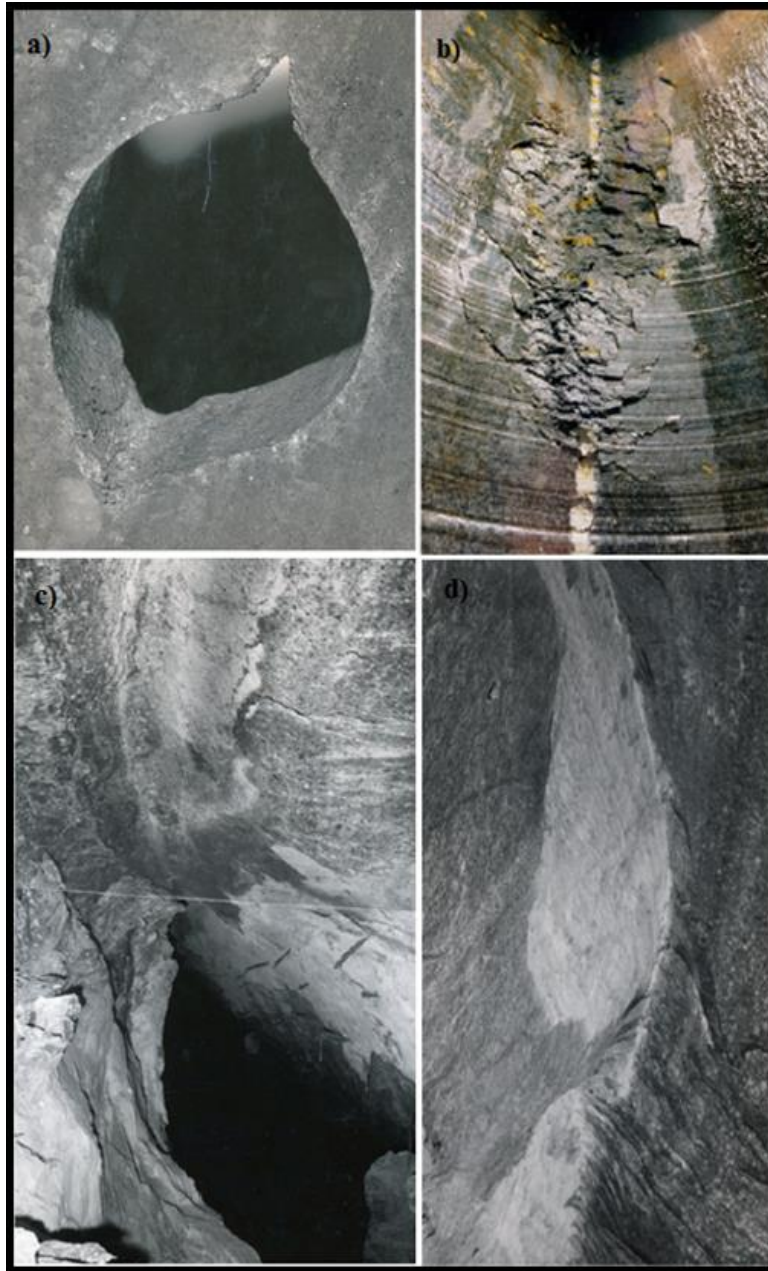
Figure 2.3.4: a) Borehole break-out b) Tunnel wall break-out. c) Micro-slabbing deterioration of crown pillar d) Initiation of micro-slabbing (Ortlepp, 1997)
