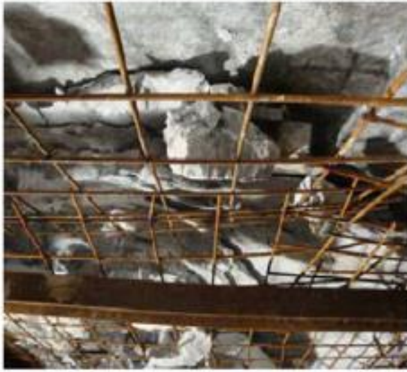
C) Phenomena of spalling in tunnel faces
