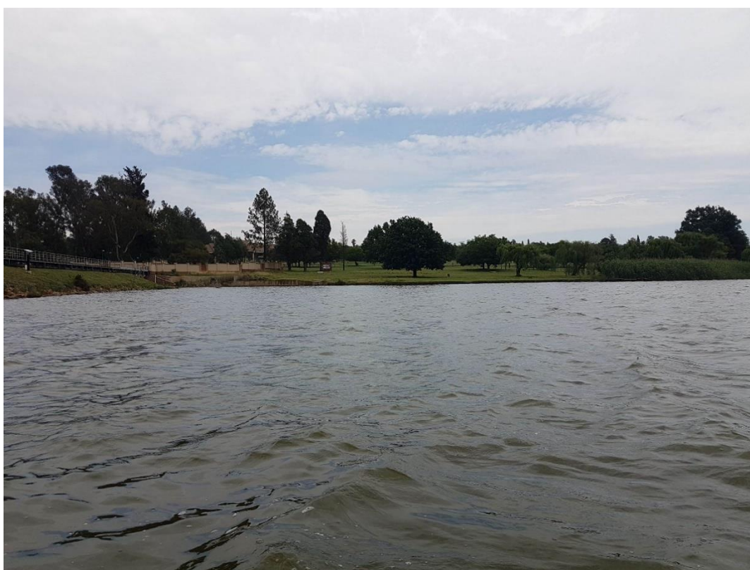
Figure 3.22: Image of van Ryn Dam taken during fieldwork in 2017
