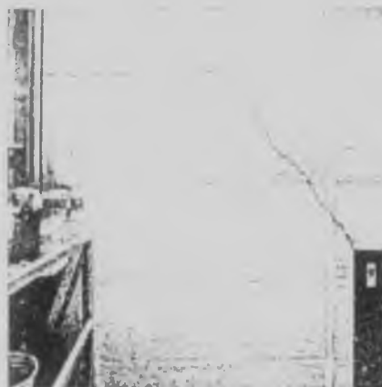
Settlement also causes cracks. Hilti's injection system ensures safe and lasting sealing of cracks.
