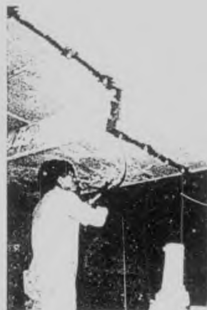
Settlement also causes cracks. Hilti's injection system ensures safe and lasting sealing of cracks.
