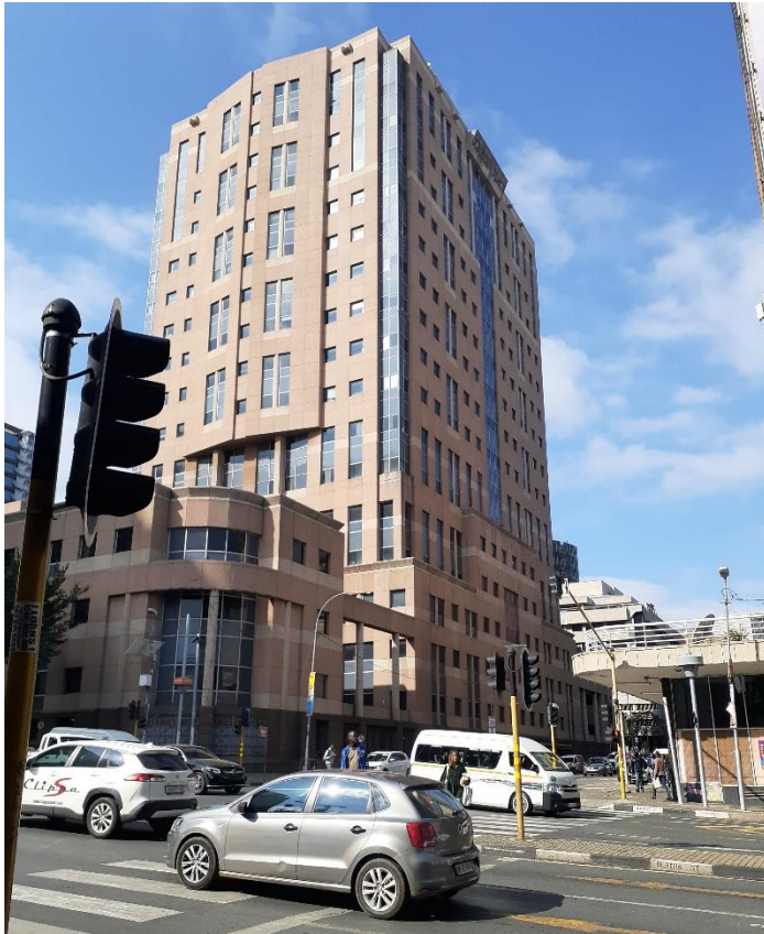
Figure 12 Dense office skyscraper. Source: Author, 2023
