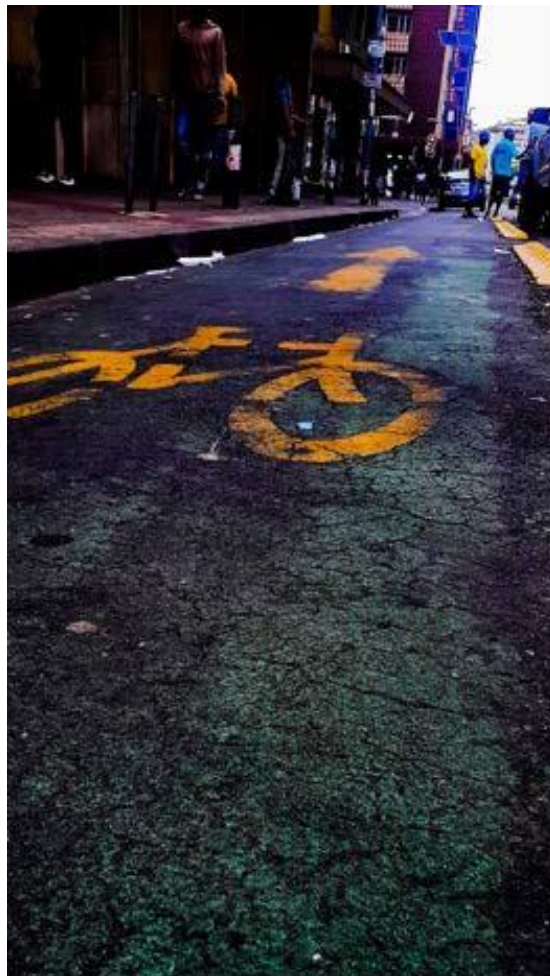
Figure 20 Cycle lane along Biccard in good condition. Source: Author, 2023
