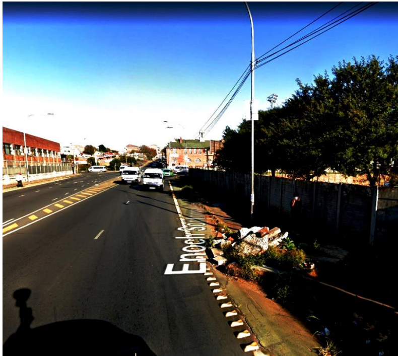
Figure 3 Rubbles and ingrown vegetation on a cycle lane along the intersection of Enoch Sontonga Avenue and Solomon Street. Source: Google Images, 2022
