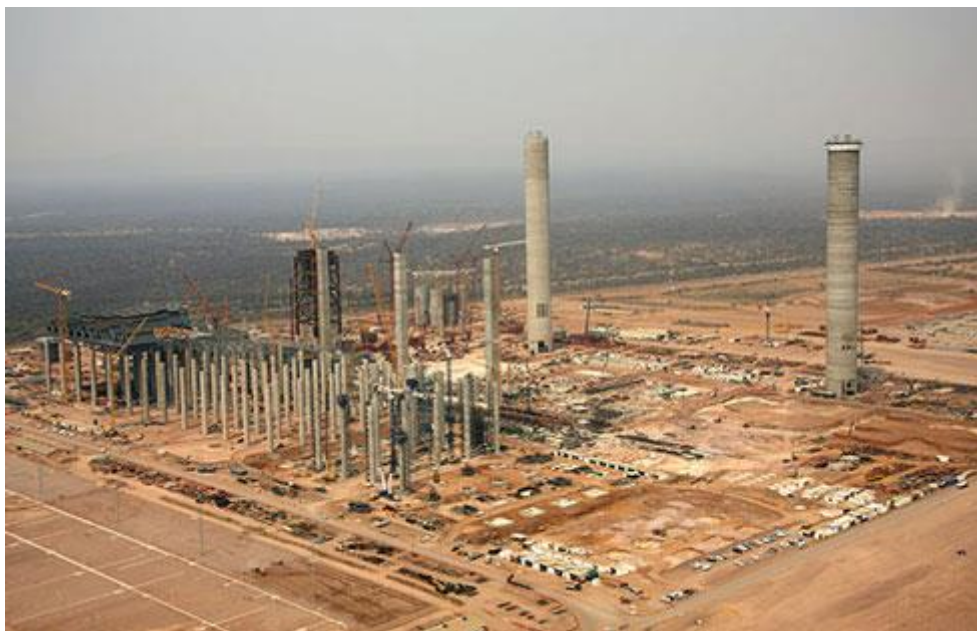
Figure 3.1: The Medupi Power Station Project at August 2011
