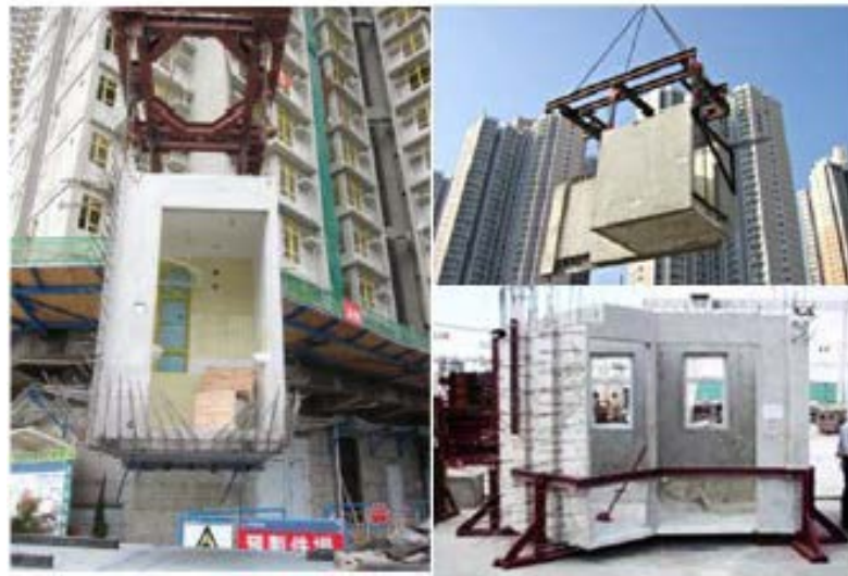
Figure 3. 4 Precast bathroom and kitchen components (Hong Kong Housing Authority, 2015 in Wong et al., 2015)
