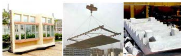
Figure 3. 3 Pre-manufactured facade, slab and staircases (Hong Kong Housing Authority, 2015 in Wong et al., 2015)
