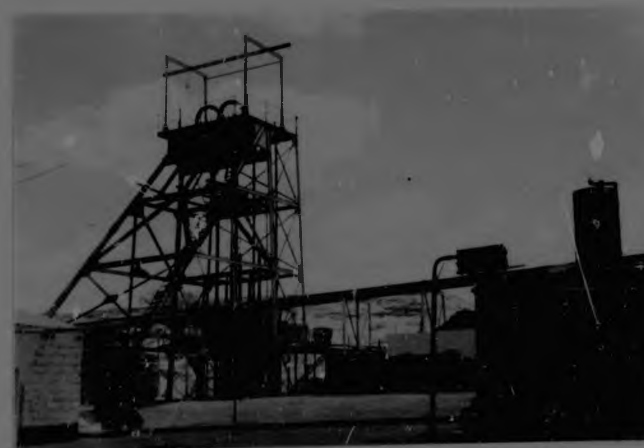
Fig. 3. Burnett Shaft headgear with rough ore-bin situated behind the compressor water-cooling tank.
