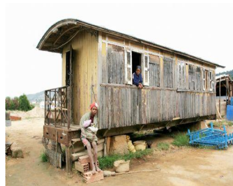
Figure 5.6. Informal settlements in Madagascar showing a house on stone columns reinforced with recycled steel in a flood prone area. Source: Copyright: UN-HABITAT (2008)
