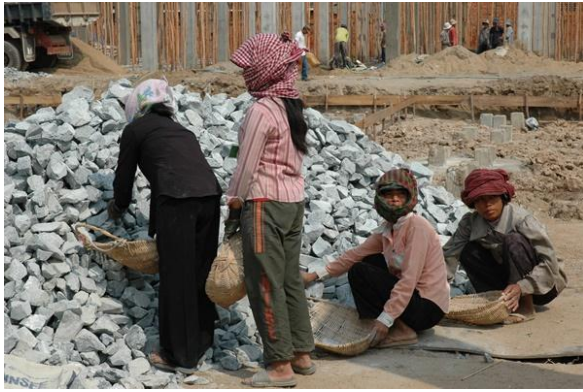
Figure 5.3. Community participation in informal settlement in Borei Keila in Cambodia. Source: Copyright: UN-HABITAT/ Mutter (2005)
