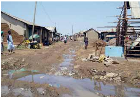
Figure 5.14. Poor infrastructure in the slums of Kisumu in Nairobi, Kenya. Copyright: UN-HABITAT (2005:21)
