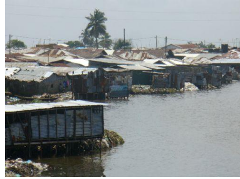
Figure 5.10. A shanty town in a slum of Monrovia showing shack development right into a waterway .Copyright: UN-HABITAT (2007)
