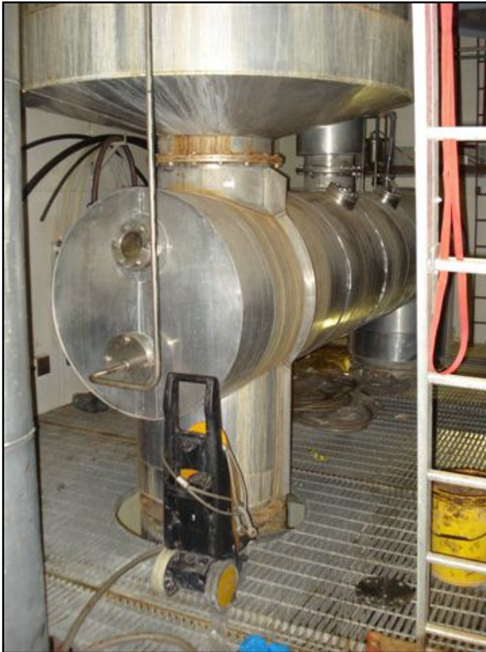
Figure 2.3 : Photograph of the upper section of the evaporator taken by the author.
