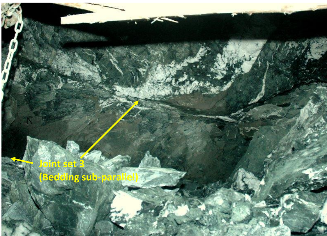
Figure 3-2 Photograph, looking east, showing 3 rd joint set at Ya Rona sub-vertical shaft (Durapraj, 2006b)
