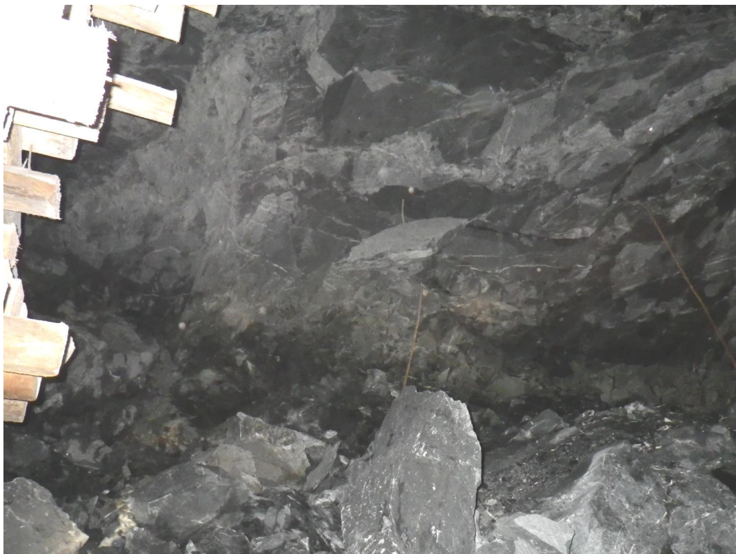
Figure 6-12 Photograph showing multiple failure surfaces of WAF which resulted in a significant fall of ground
