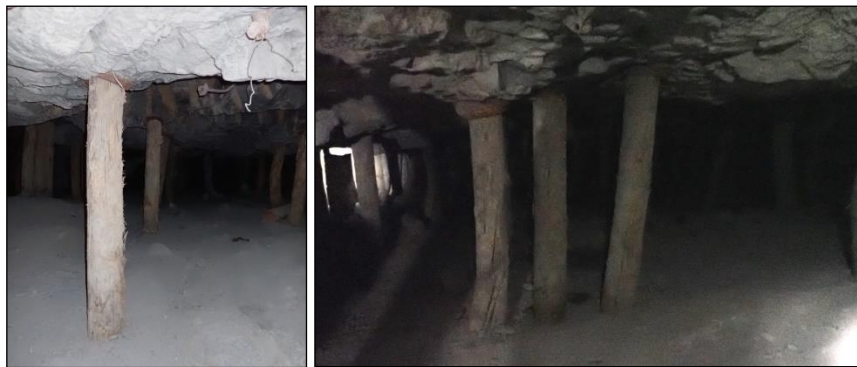
Figure 4.24: Mine pole support in short panel.
