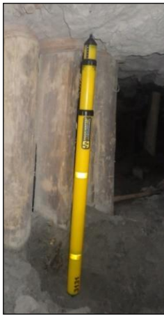
Figure 2.10: Closure logger installed in a stope panel.
