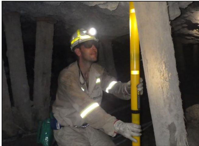
Figure 3.2: Closure logger installation by the author.
