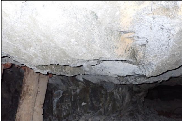
Figure 4.6: Hangingwall condition around the crush pillar.
