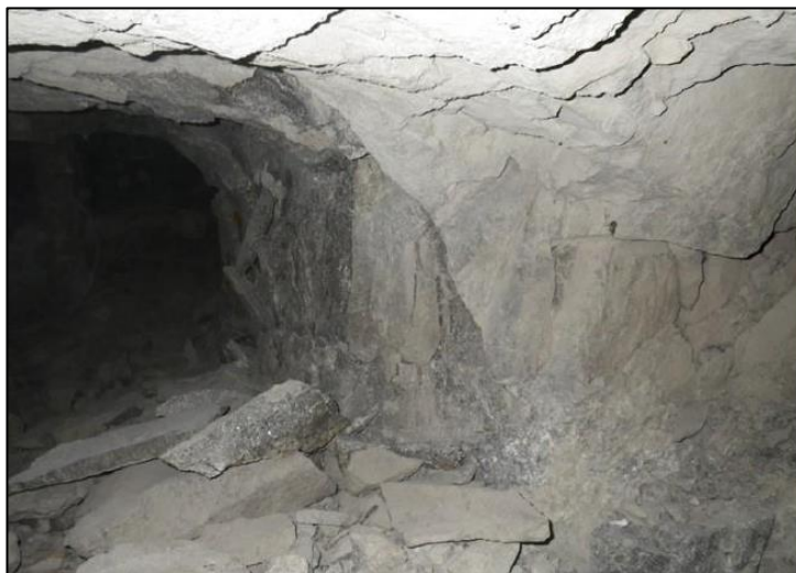
Figure 3.8: Crush pillar scaling at N15 Level.
