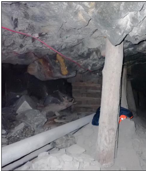
Figure 4.1: FOG along C-packs prevented further unravelling.
