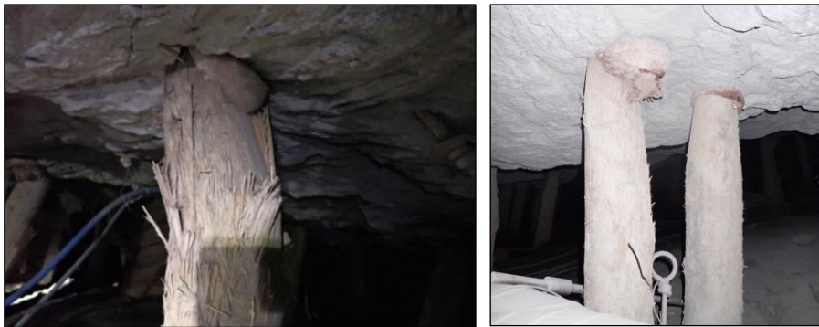
Figure 4.22: Pencil sticks showing rapid yielding.
