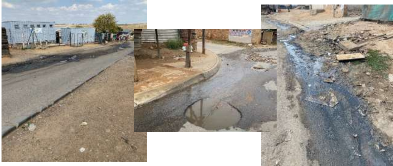
Figure 4.3 Mixed quality of terrain in the community with areas of potholes, overflowing sewage and rubbish
