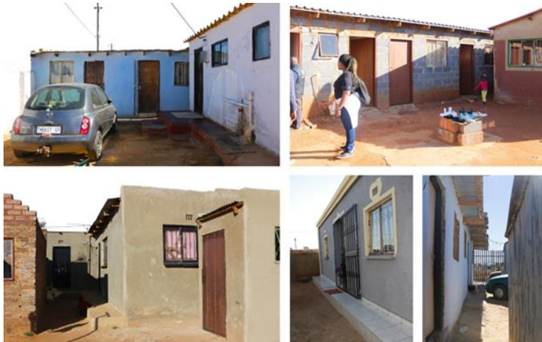
Figure 4.1; Backyard dwelling built by landlords in Bram Fischerville (Selepe, 2016).
