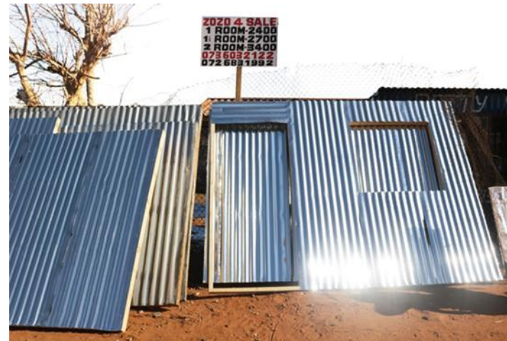
Figure 2.1; Zozo shacks advertised in front of where they are made in Bram Fischerville. (Selepe, 2016).
