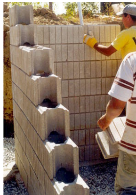
b) Dry-stacking Azar blocks
