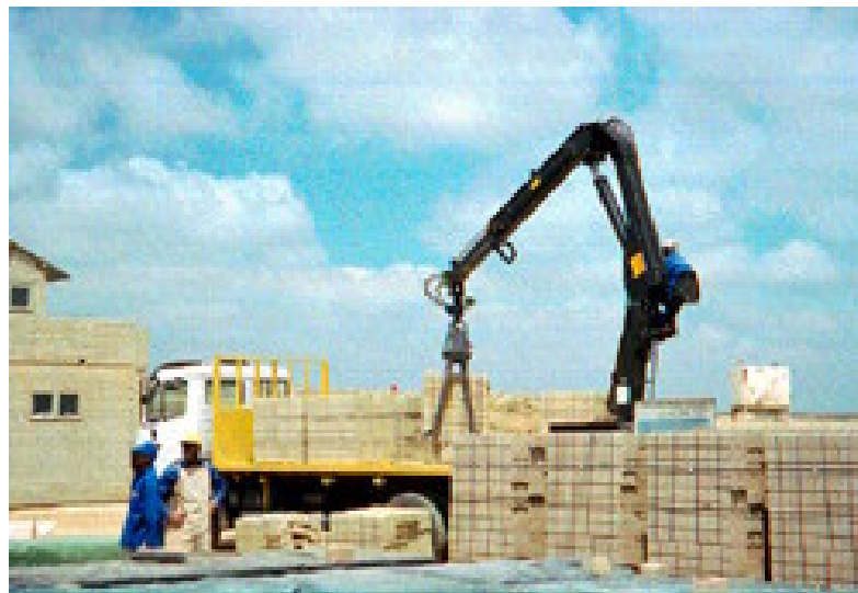
Figure 2.29 Delivering of the blocks in pallets
