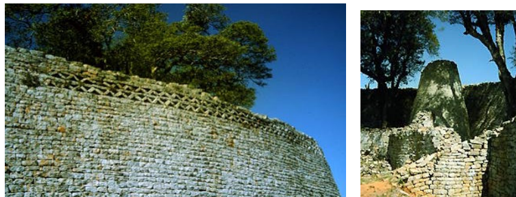
a) Dry-stack fencing wall
