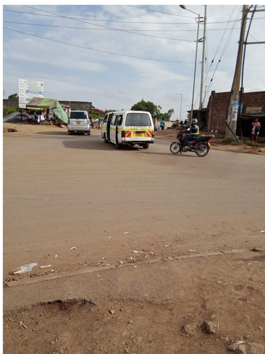
FIGURE 4 Photo of the built environment: roads without signposts, markings, and speed controls as well as and drainages without covers (Taken by a PWD).
