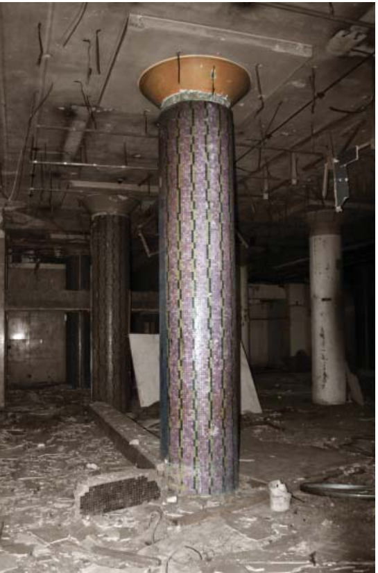
Figure 71 and Figure 72: Photograph showing the internal degradation and violation of the CNA Building, where the only remaining detail is the columns cladding mosaic.
