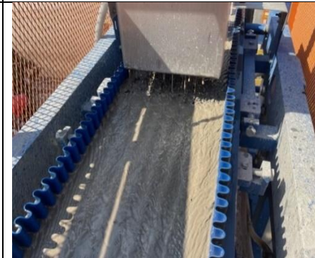
Magnet bed full of slurry..
