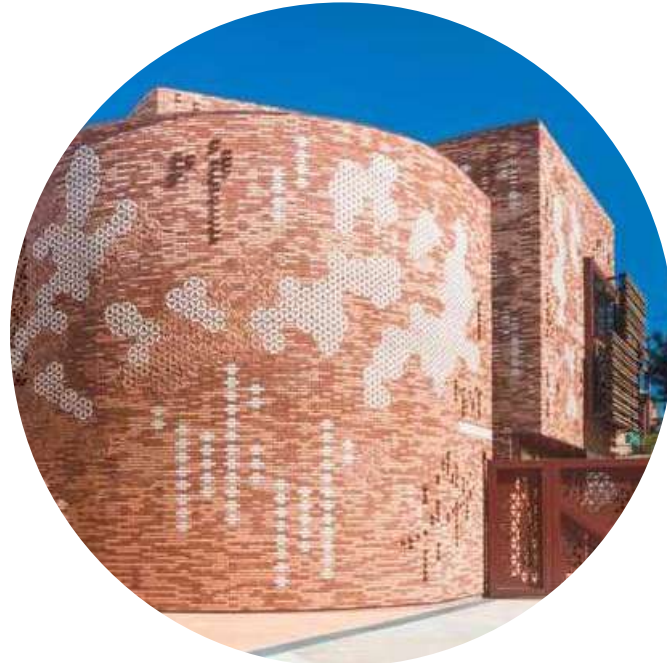
Fig 200. Textured Brick Facade. Miralles Tagliabue (2019)
