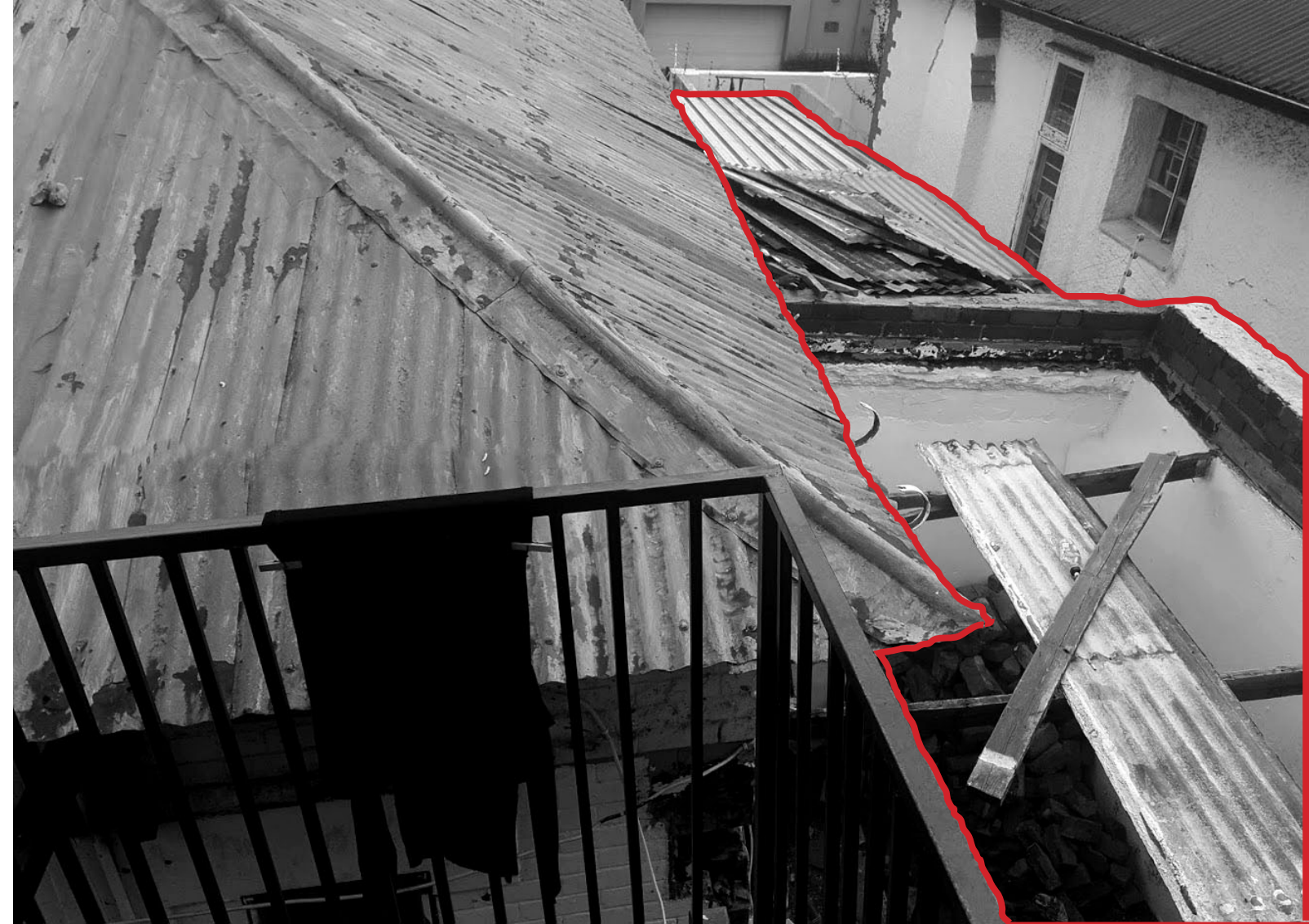
Fig 58. View from second floor of backyard structure showing attachments to original bungalow and neighbouring bungalow. Authors Own (2018)
