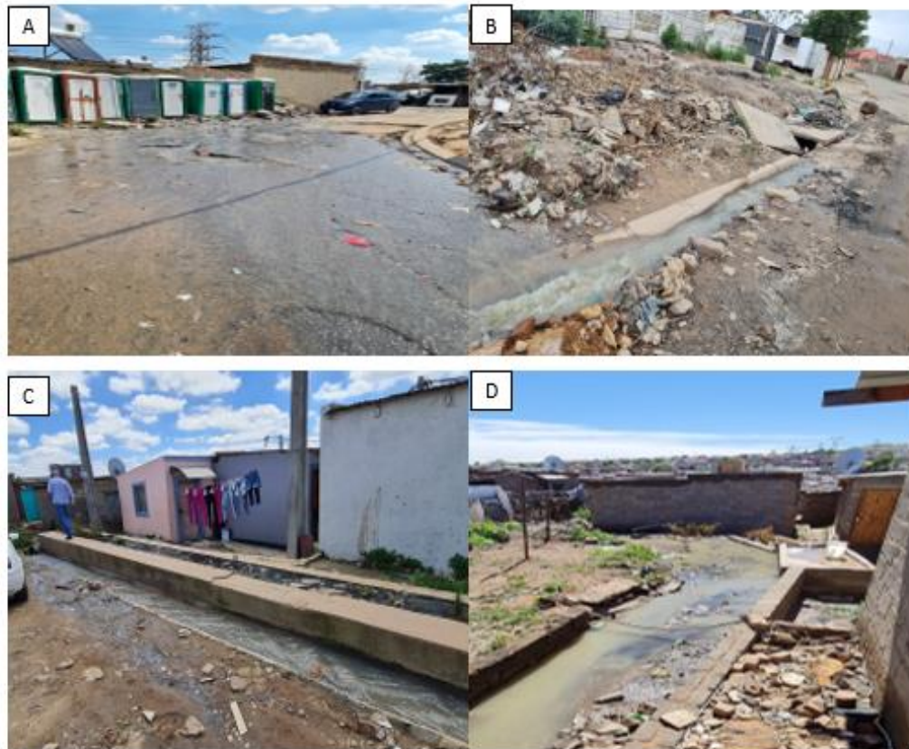
Figure 40: A sequence of water flows ultimately result in the flooding and destruction of CW2.
