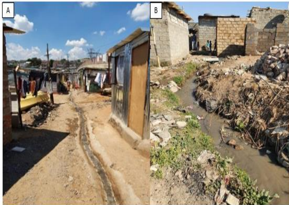
Figure 24: Developed and paved gully in Setswetla (A). A gully that has turned into a bigger stream overtime in Silvertown (B).
