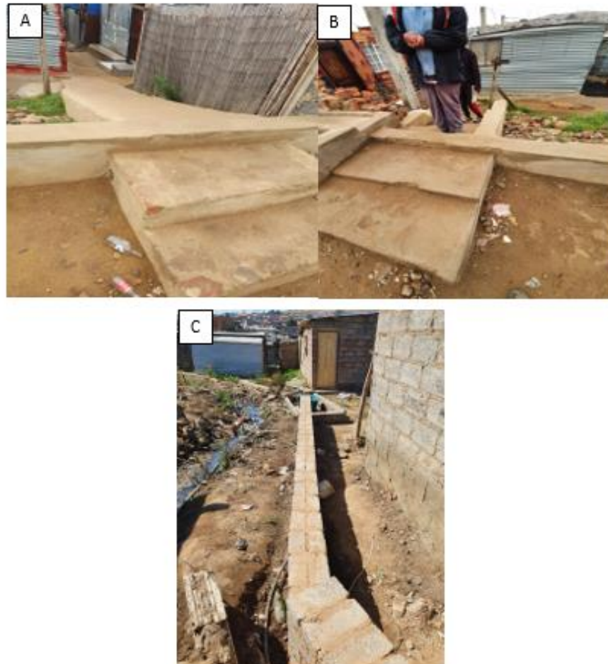
Figure 35: A photo showing a ramp (A) staircase (B), and wall (C) built in Silvertown.
