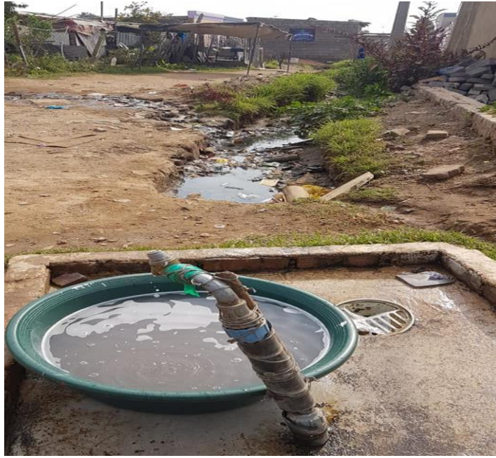
Figure 14: A broken tap at the site of CW1 before building.
