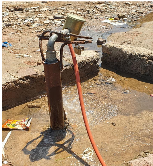
Figure 15: A communal tap with a lock placed around the tap.
