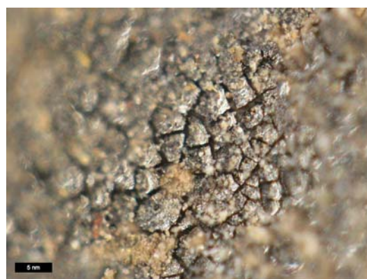
Figure D.49: 1= Micrograph of the cracked stone surface on SBL10. Magnification 200.
