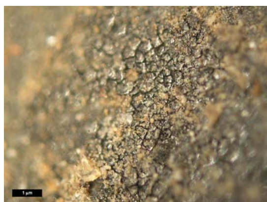
Figure D.48: 1= Micrograph of the cracked stone surface on SBL10. Magnification 100.
