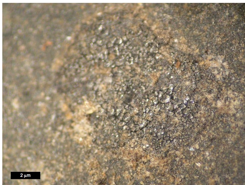
Figure D.47: 1= Micrograph of the cracked stone surface on SBL10. Magnification 50.
