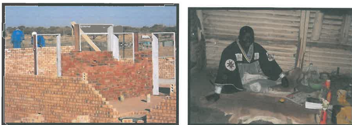
Figure 3-5: Pictures showing health facilities in Smash Block
