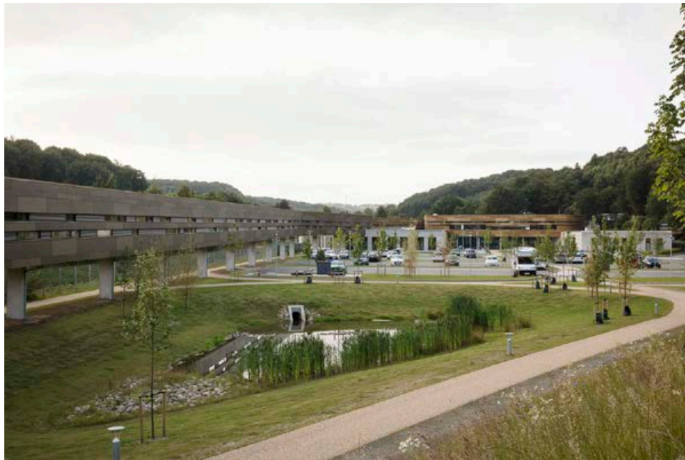
Fig 6.5 - Landscaped entrance to facility
