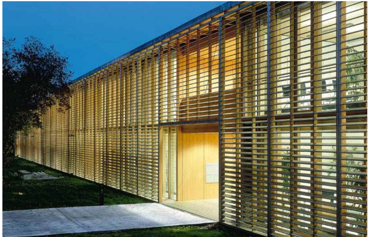
Fig 6.8 - Entrance to facility
