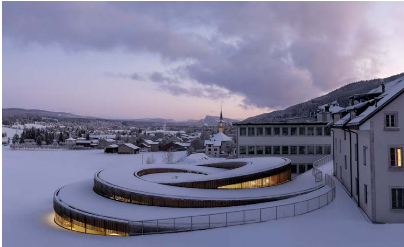
Fig 6.11 - Exterior View of Building
