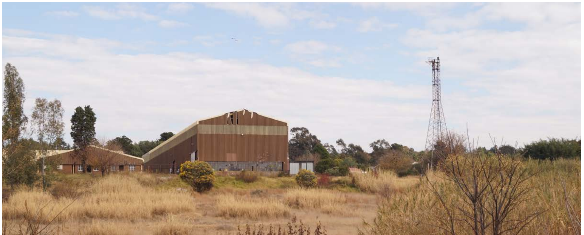
Fig 4.4 - View of existing structures and landscape
