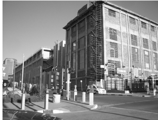
Turbine Hall. Newtown, Johannesburg
