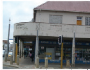
Image 4 :good street interface with commercial ground floor and flats above
