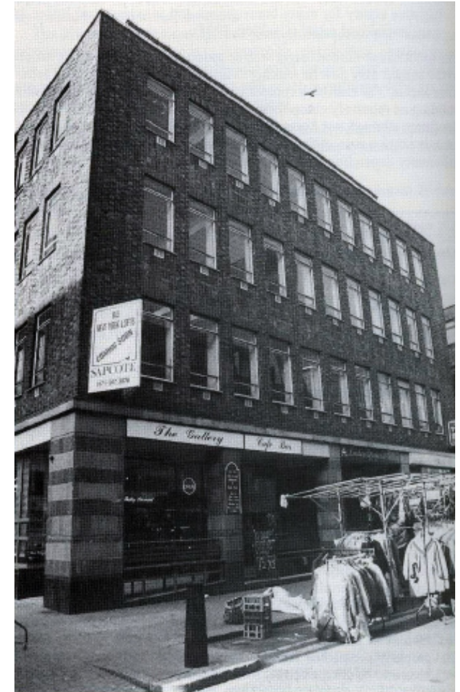
Dorrington House, Leather Lane, London Offices over shops (originally to be converted for residential use) (Coupland 1997: 120)
