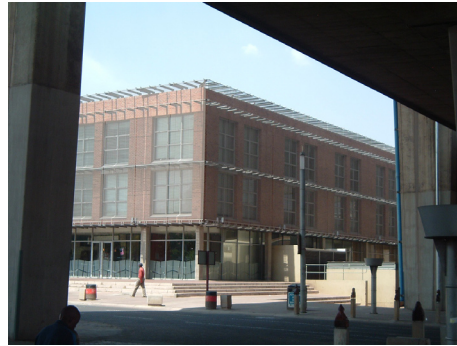
7) View looking under the highway towards Turbine Hall
