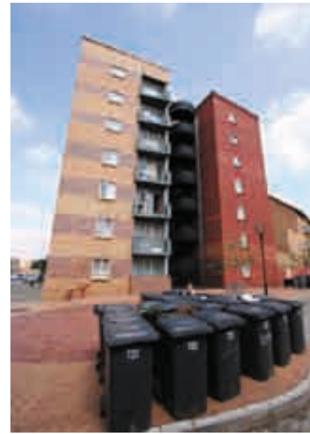
Open stairwell at Legae which gives visual links for the residents to their surroundings (Existens Maximum 2008: 60)
