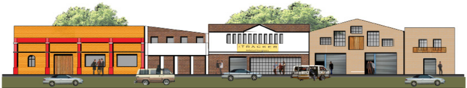
Existing buildings on Bree Street
