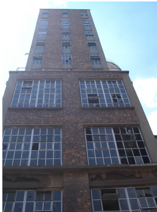
Old industrial building. Newtown, Johannesburg
