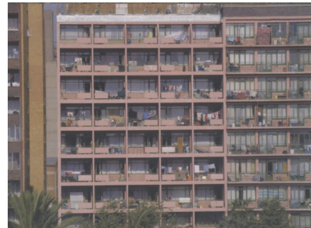
Flats in downtown Johannesburg (Burdet, Sudjic 2007: 197)
