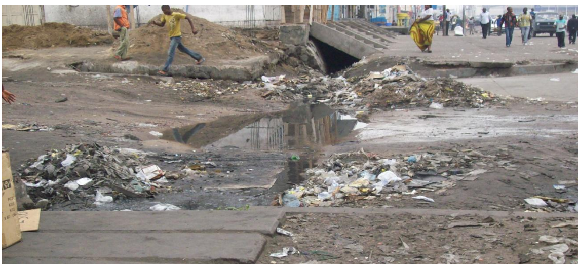
Figure 2: Divested Infrastructure in Kasavubu corner Victoire Street, in KLM July 2009
