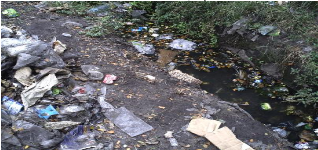
Figure 12: Open gutter blocked with ashes solid wastes in the corner Huillerie and Kato Streets in the west of KLM, July 2009
