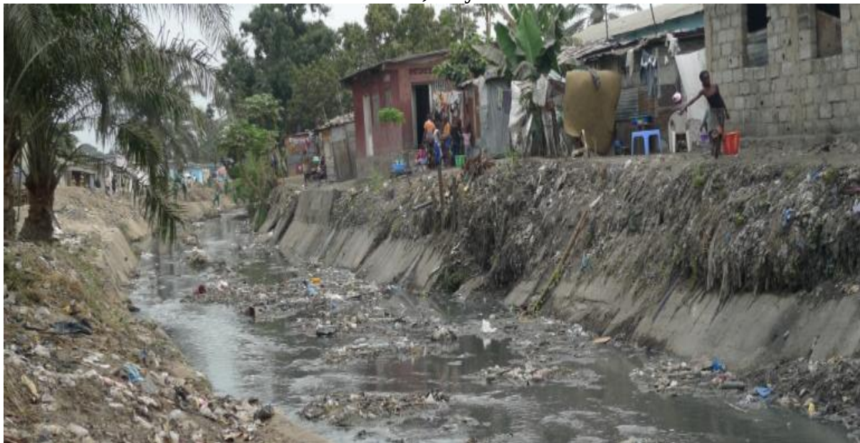
Figure 10: Drainage Channels at Bitshaku-Tshaku River Next to 24 November Stadium, July 2009
