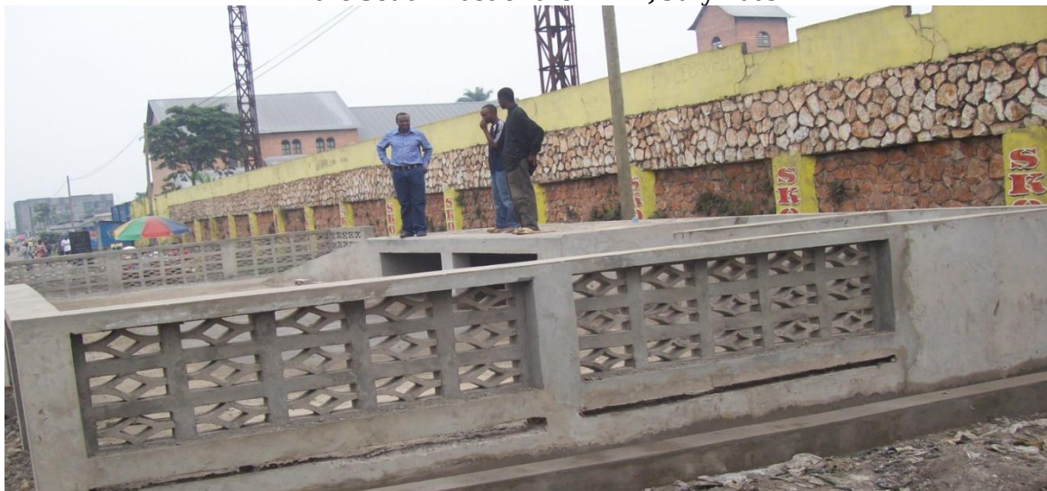
Figure 28: PAUK's Construction of a Formal Disposal Site outside St Pierre Stadium in the South-East of the KLM, July 2009
