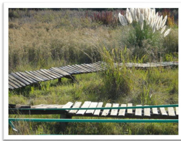
Figure 5.4 The wooden structures are raised over the wetland to prevent cycling through the wetland and causing damage to the wetland (Author: 2008)
