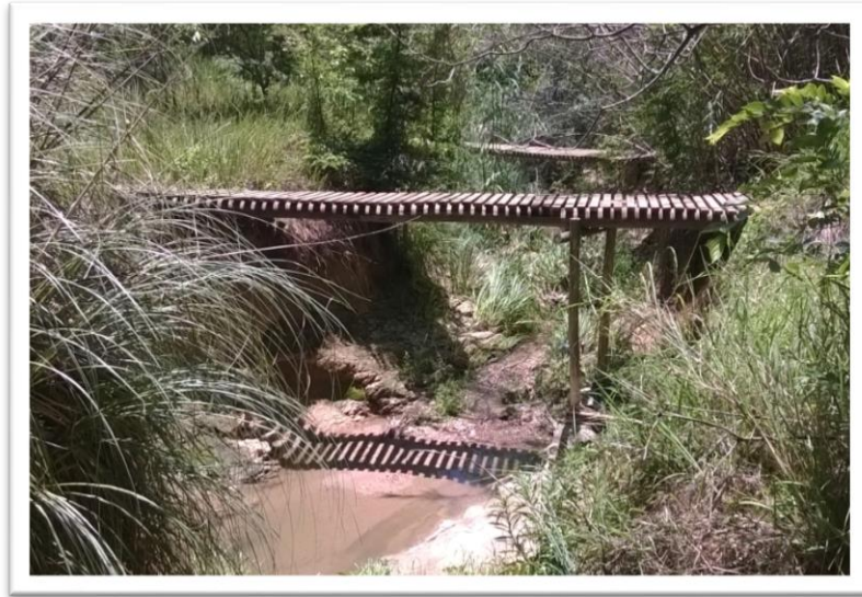
Figure 5.8 Example of ongoing erosion on the site (Author, 2014).
