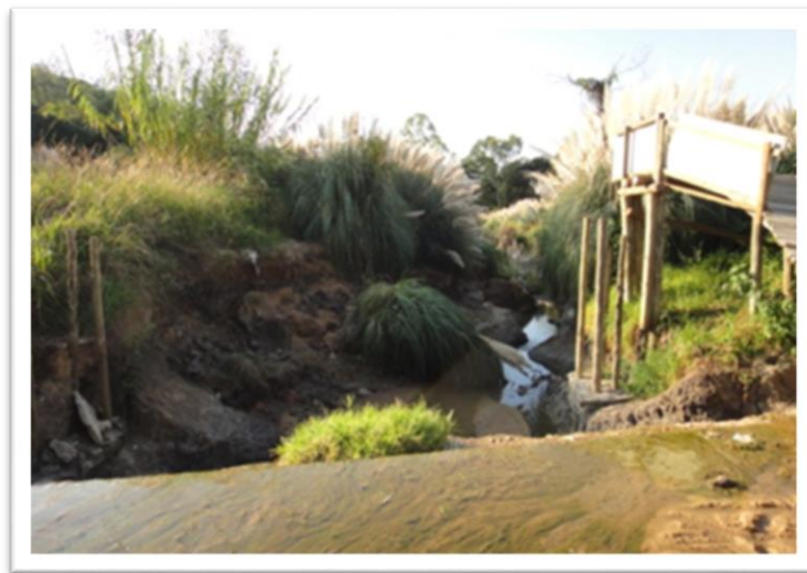
Figure 5.6 Severe gully erosion on the site downstream of the “widened” section of the stream. (Author: 2012)
