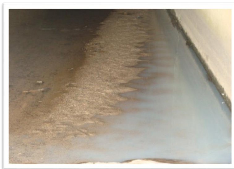
Figure 7-10 Liesbeek River: Milky discharge in stormwater outlet (Author: 2013)
