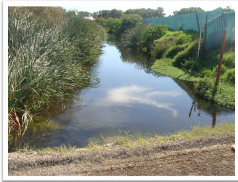
Figure 7-2 Macassar: Upstream showing left bank (Author: 2013)
