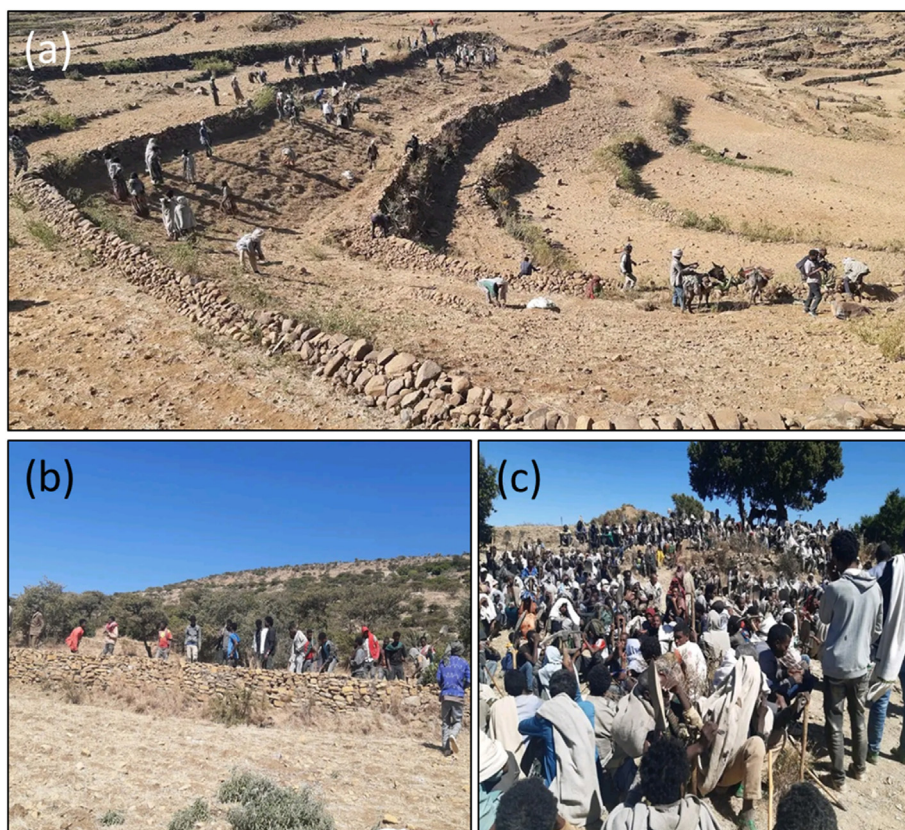
Fig. 7. Soil and water conservation practice at Dejen village, Enderta District, January 2023. (a) Construction of stone bunds on sloping land; (b) Maintenance of destroyed stone bunds; and (c) After soil and water conservation work, farmers gathered to evaluate the performance (Source: Photos taken by authors).
