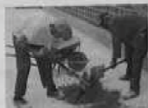
Ernest and Orbit mixing cement and sand
