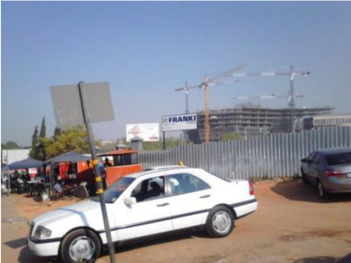
Figure 74 : Photograph of the building of the Growthpoint development off West Street, Sandton.
