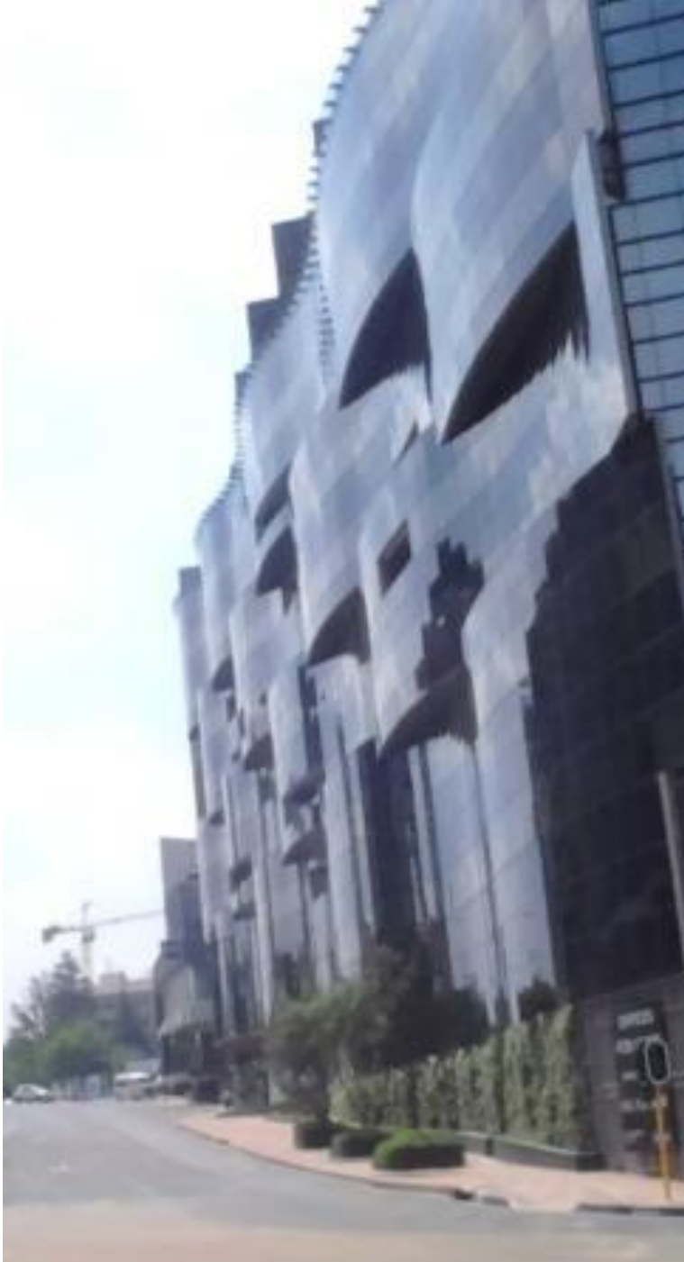
Figure 9 : A view of a façade on West Street
