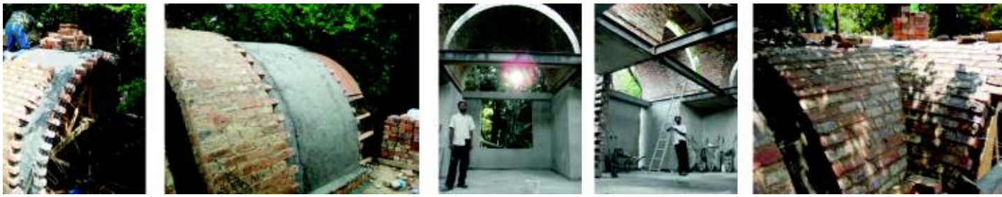
177 - Example of a groin vault built locally, designed and built by Lewis Levin Architect (Images Courtesy of Nick Mallandain)
