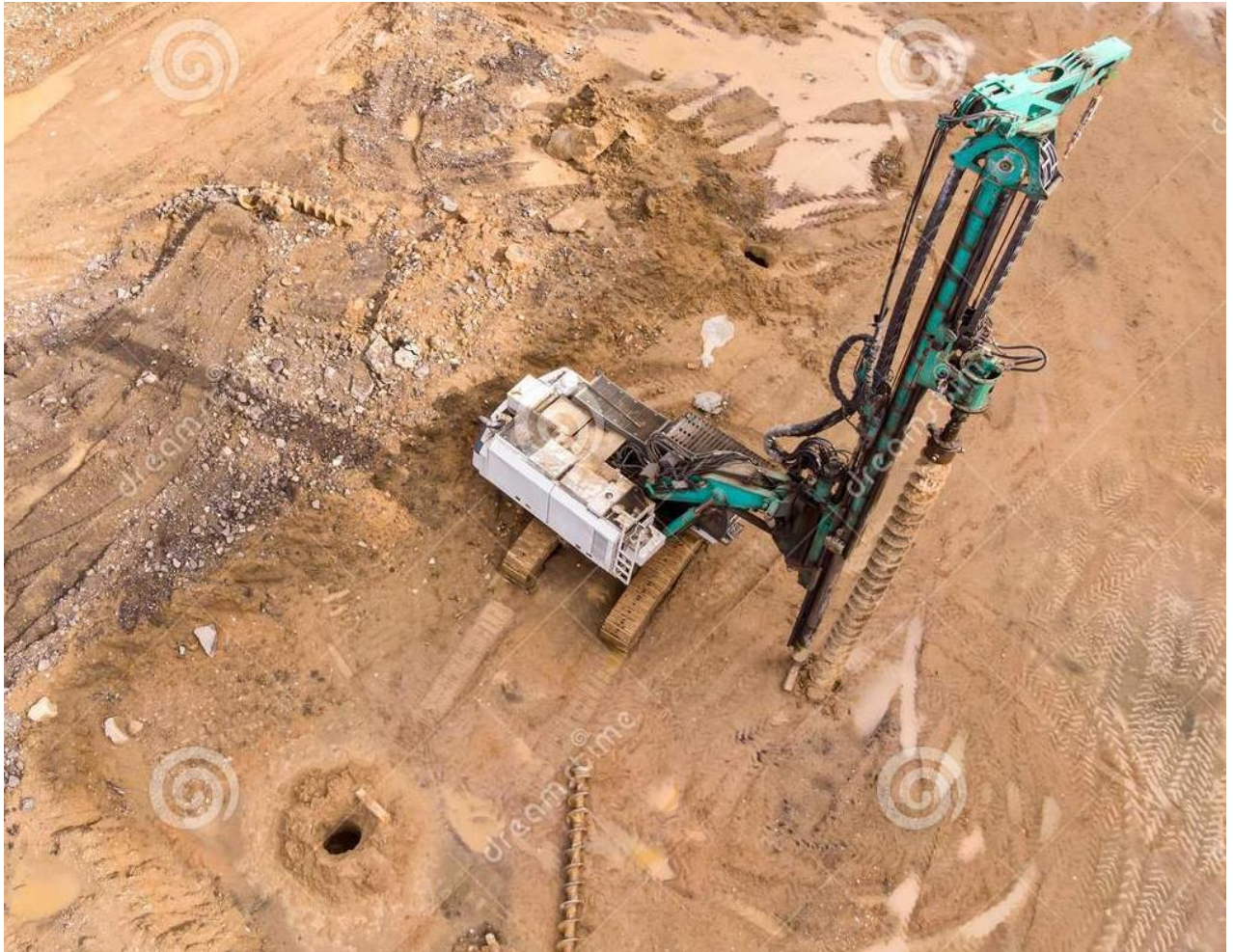
Figure 2. Drilling machine in operation (iStock, 2022)
