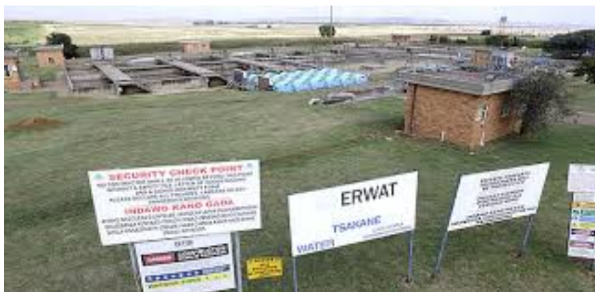
Fig 3.5 ERWAT wastewater water treatment work, Ekurhuleni South Africa
