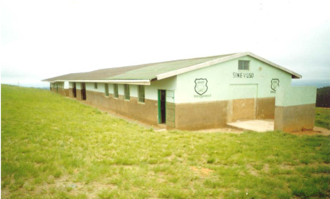
Figure 1.3 Sinevuso Secondary School
