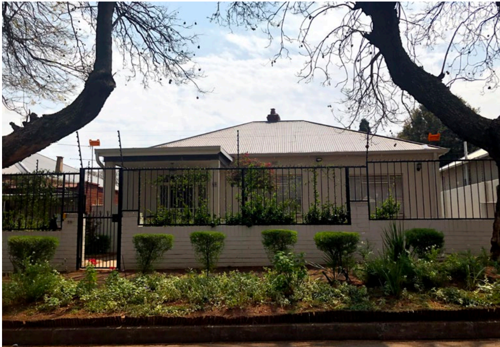
Figure 106: Low Rise Residential Building with Sheetting on the Roof(Baart, 2020)
