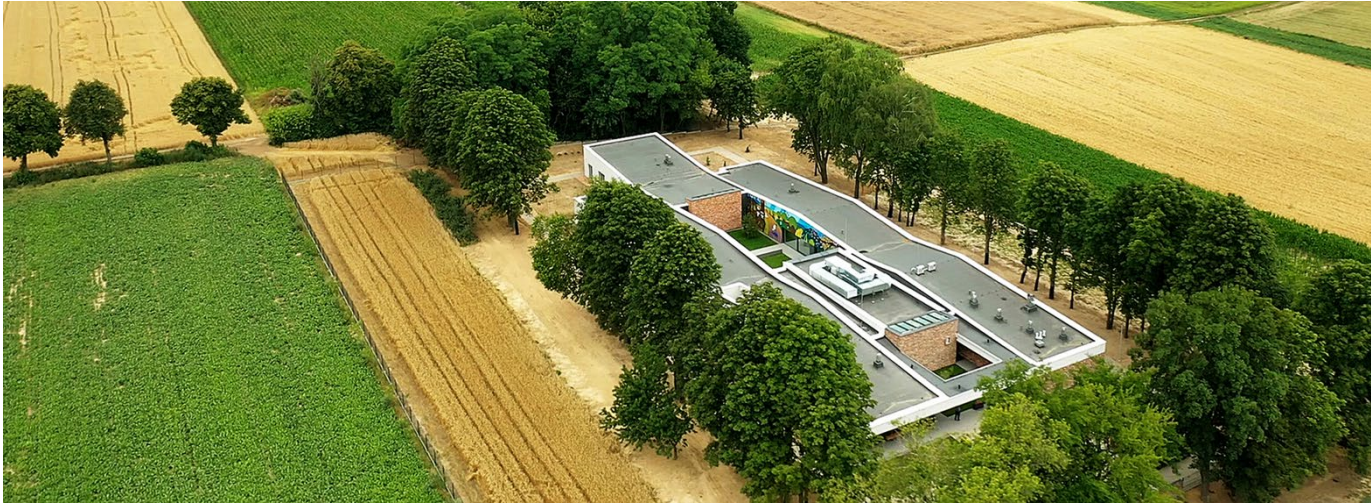
Figure 52: Aerial Image of Home for the Homeless (One Light Studio 2019)
