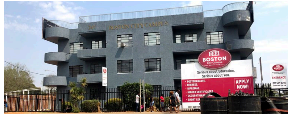
Figure 104: Some Bulky Buildings are found which Celebrate Balconies (Baart, 2020)
