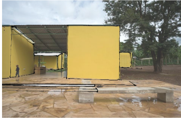
Figure 61: External View of KWIECO Shelter (Ilonen 2015), Illustration (Baart, 2020)
