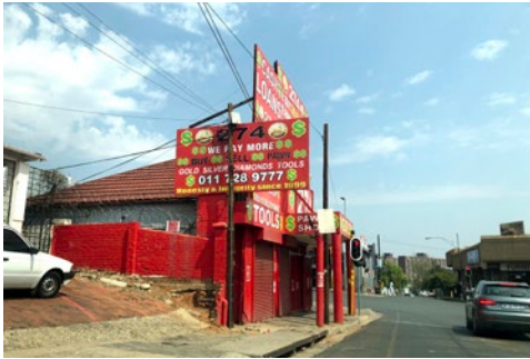
Figure 91: Corner Building (Baart, 2020)
