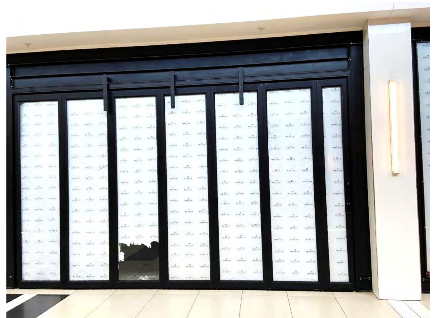
Figure 33: Covered Windows of Vacant Shops
