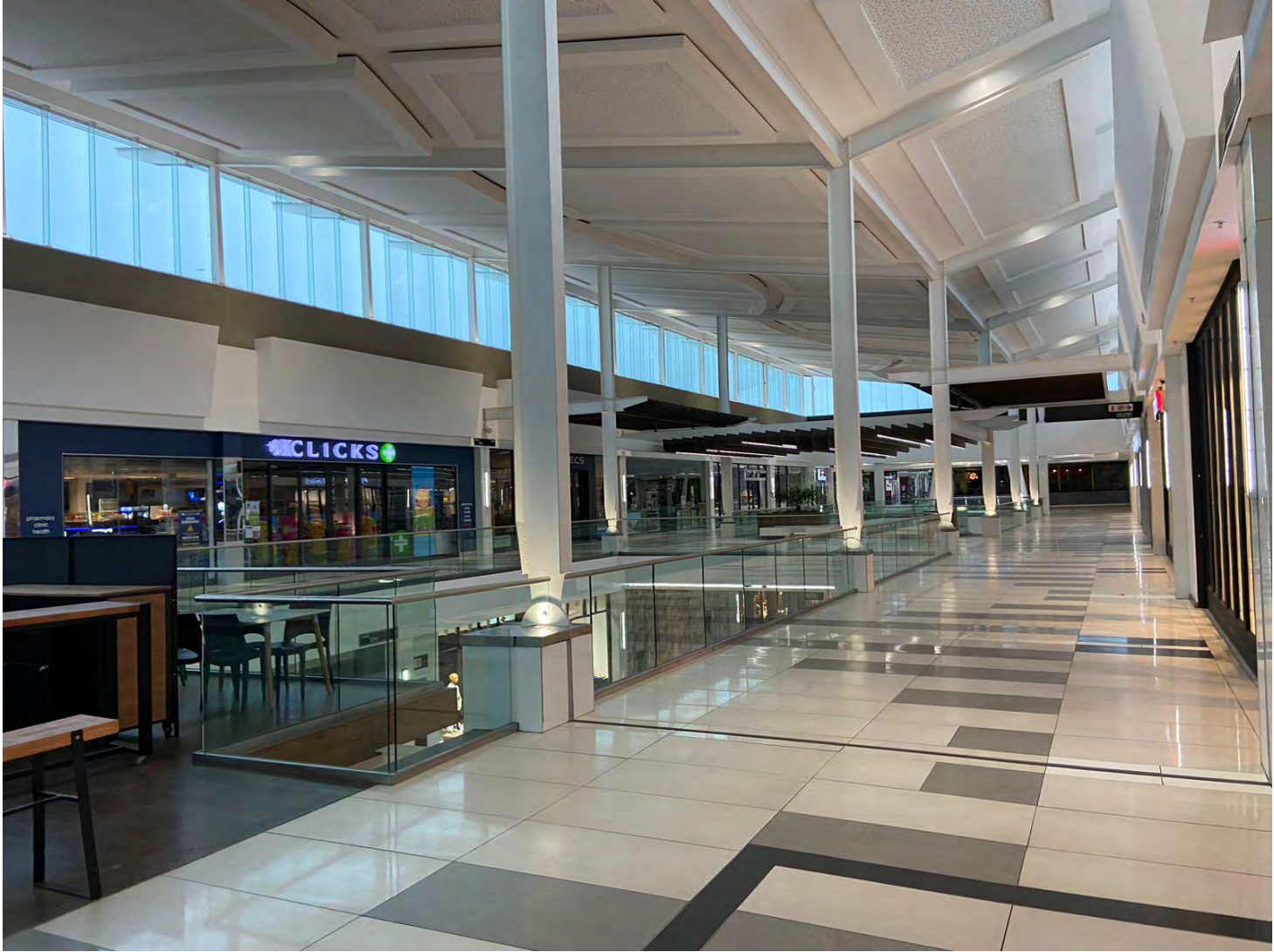
Figure 54: Skylights along the roofline
