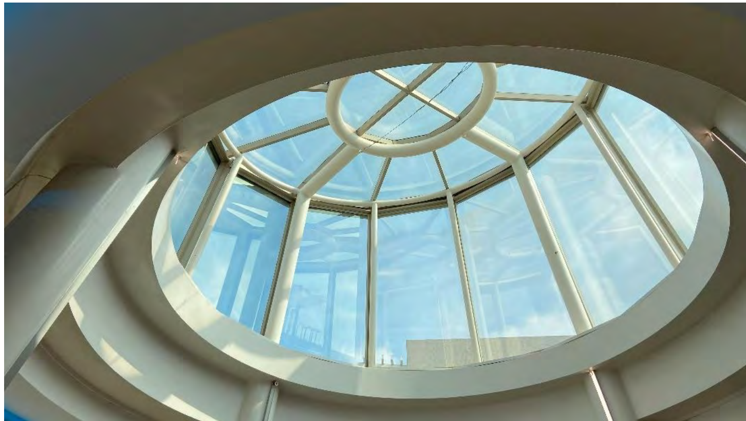
Figure 55: Skylight at walkway intersection
