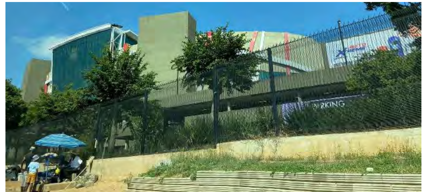
Figure 46: Edge Condition Along Lois Avenue
