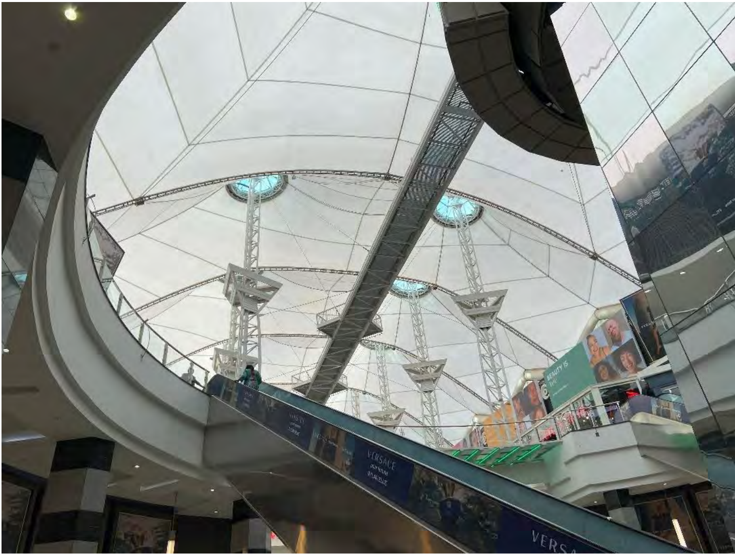
Figure 63: Tent covering the Grand Hall
