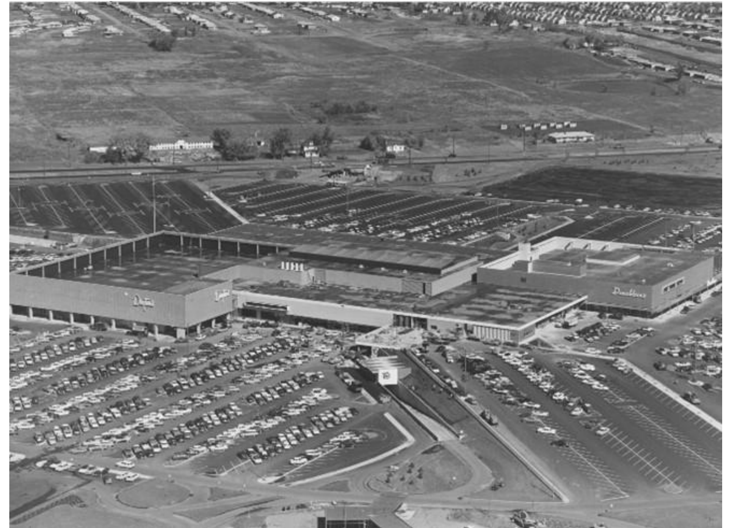
Figure 15: Exterior of Southdale Centre Mall (City of Edina, Minnesota, 2018)
