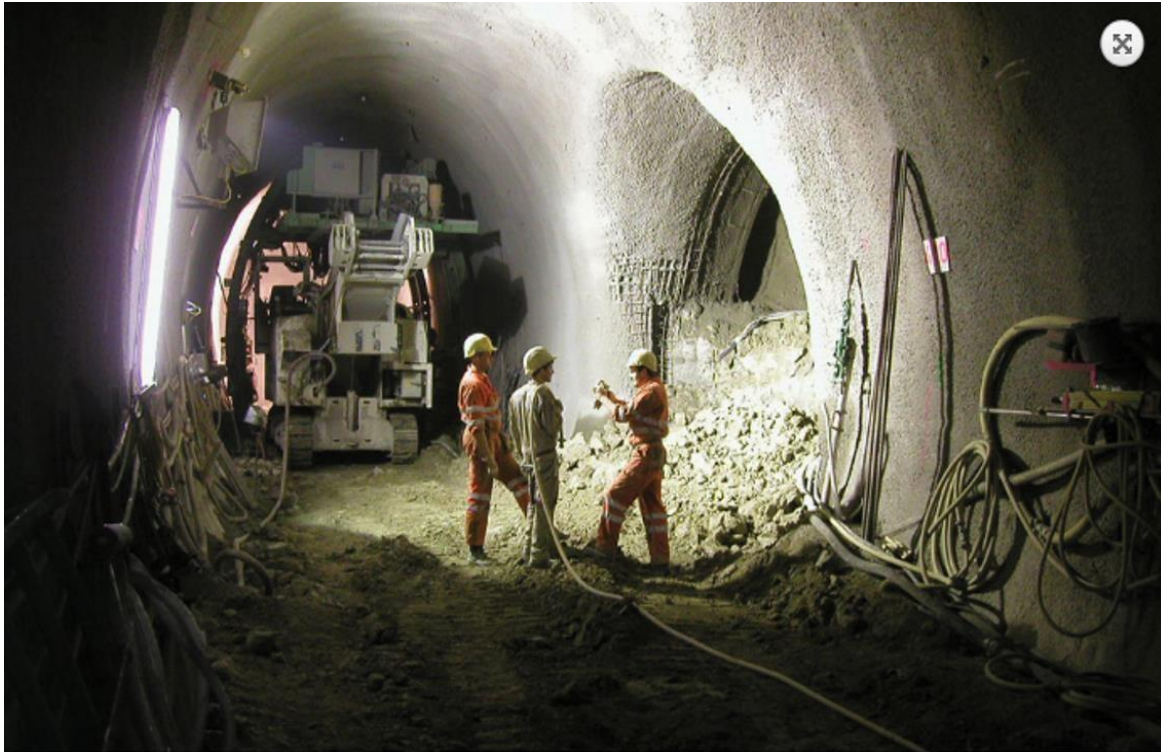
Figure 18: Spraying of shotcrete on tunnel walls (Anon., n.d.)
