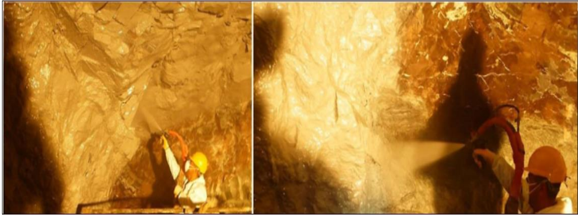
Figure 19: Application of TSL on tunnel walls (Anon., n.d.)
