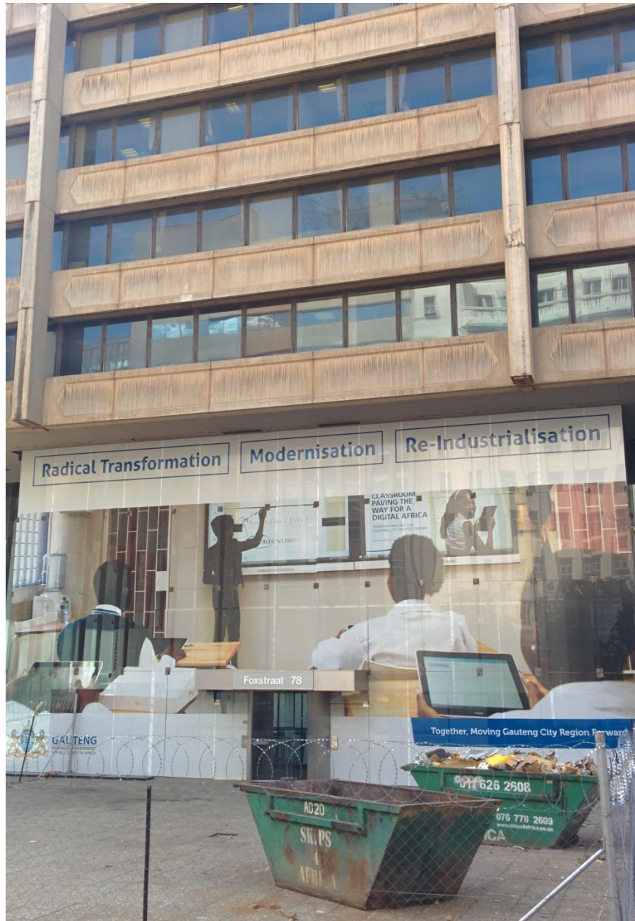
Figure 8. Scaffolding in front of the former Standard Bank headquarters on Main Street.
