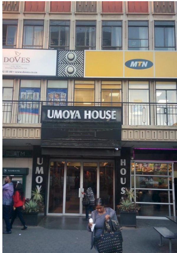
Figure 18. The façade of two buildings owned and managed by Gerald Olitzki's company OPH, located on Loveday and Rissik Street respectively, both in Marshalltown.
