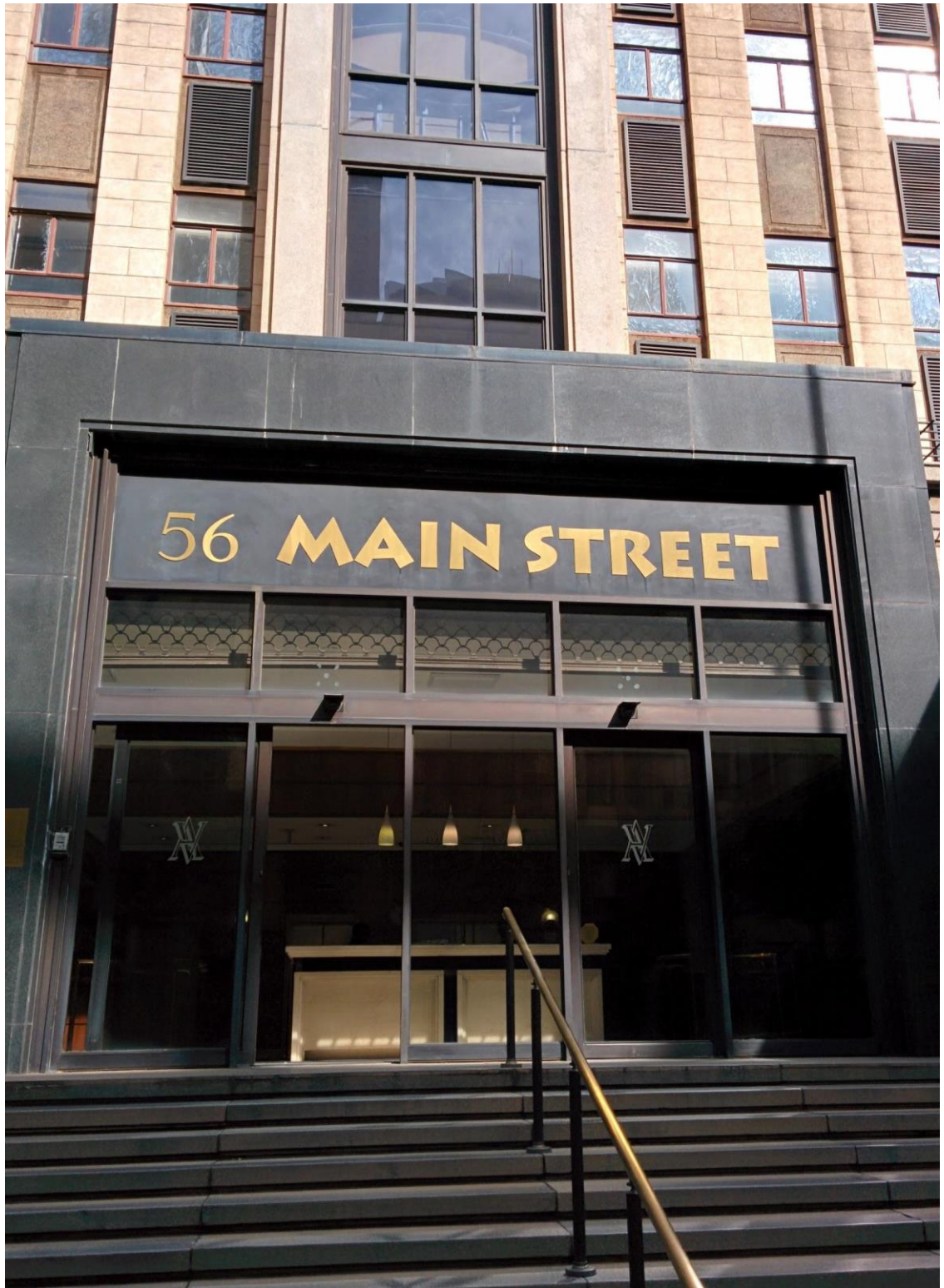
Figure 19. Building owned by the Anglo American Corporation on Main Street.
