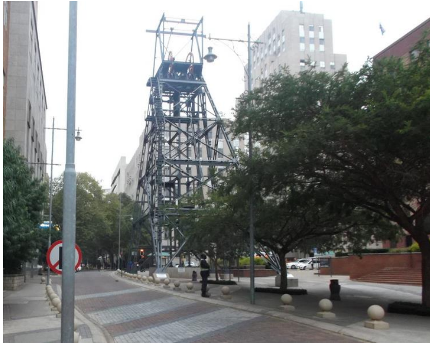
Figure 11. Mining headgear at the corner of Main and Simmonds Street.
