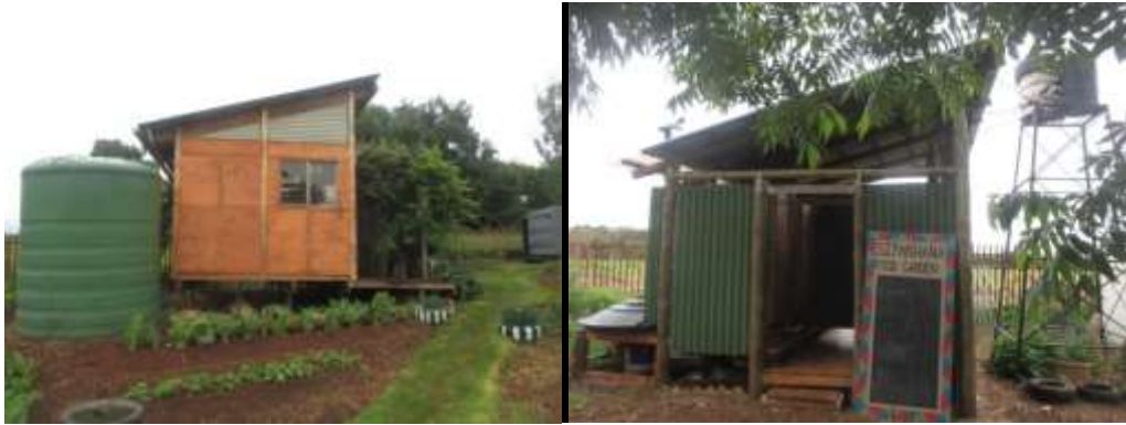
Figure C.0-4: The eco-office and toilet (source, author)
