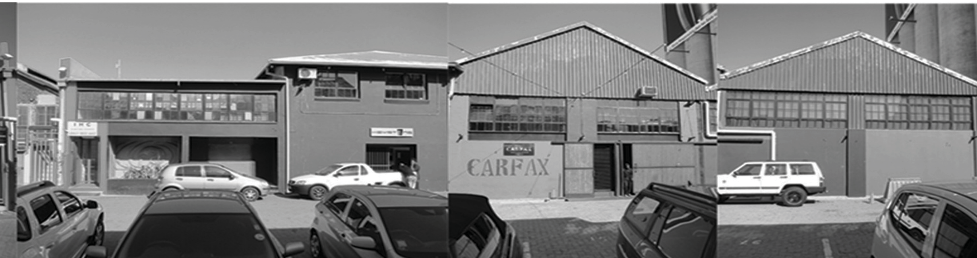
The buildings that are proposed to be demolished view from the north sidings
