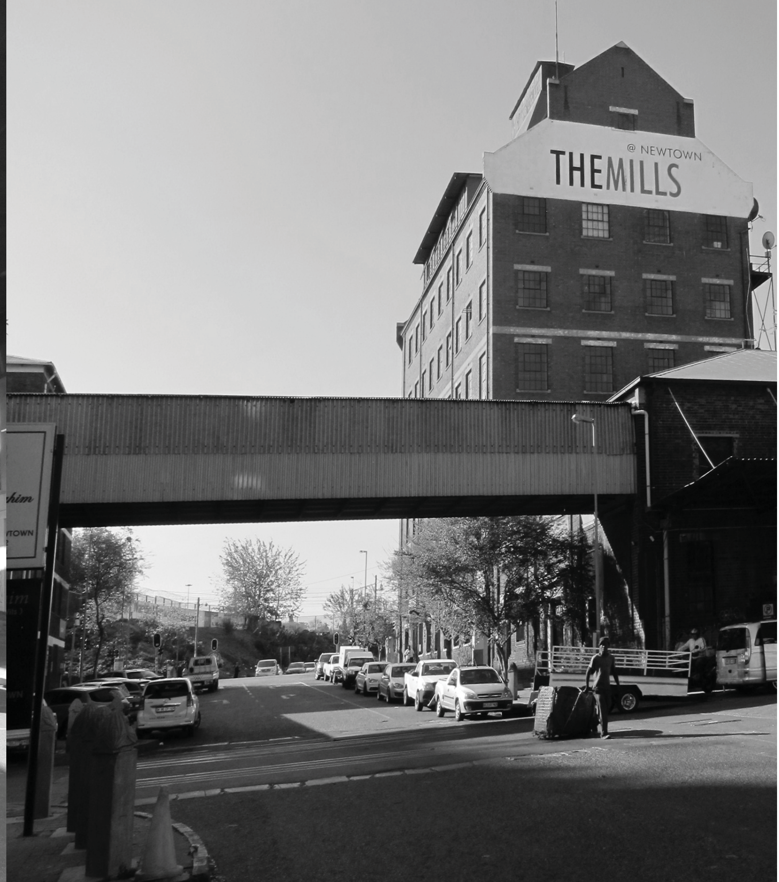
A bridge , a literal connection spans Quinn street. A Roof covers the entrance of the east north sidings (originally used to keep goods dry during the loading process ) and forms an entrance threshold. (Authors own work ,2016)
