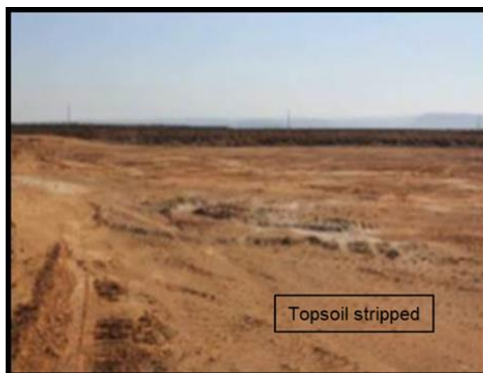
Figure 3-1: Topsoil removed for scanning using GPR (Tweefontein Opencast Colliery, 2013; van Schoor, 2013)
