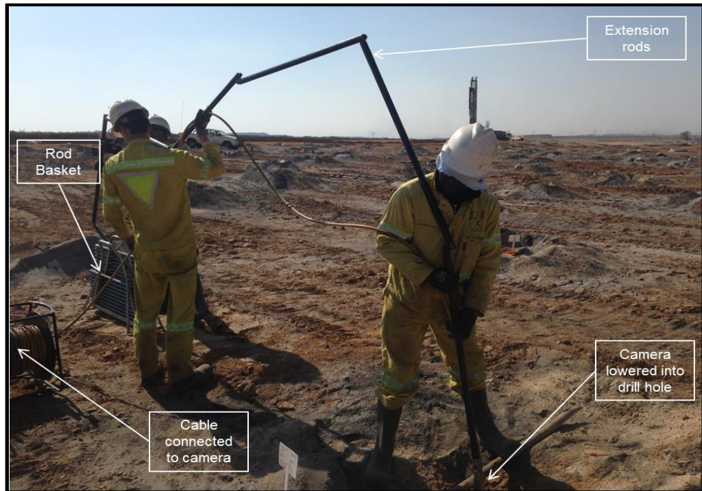
Figure 3-11: CALS Tool being lowered into a hole
