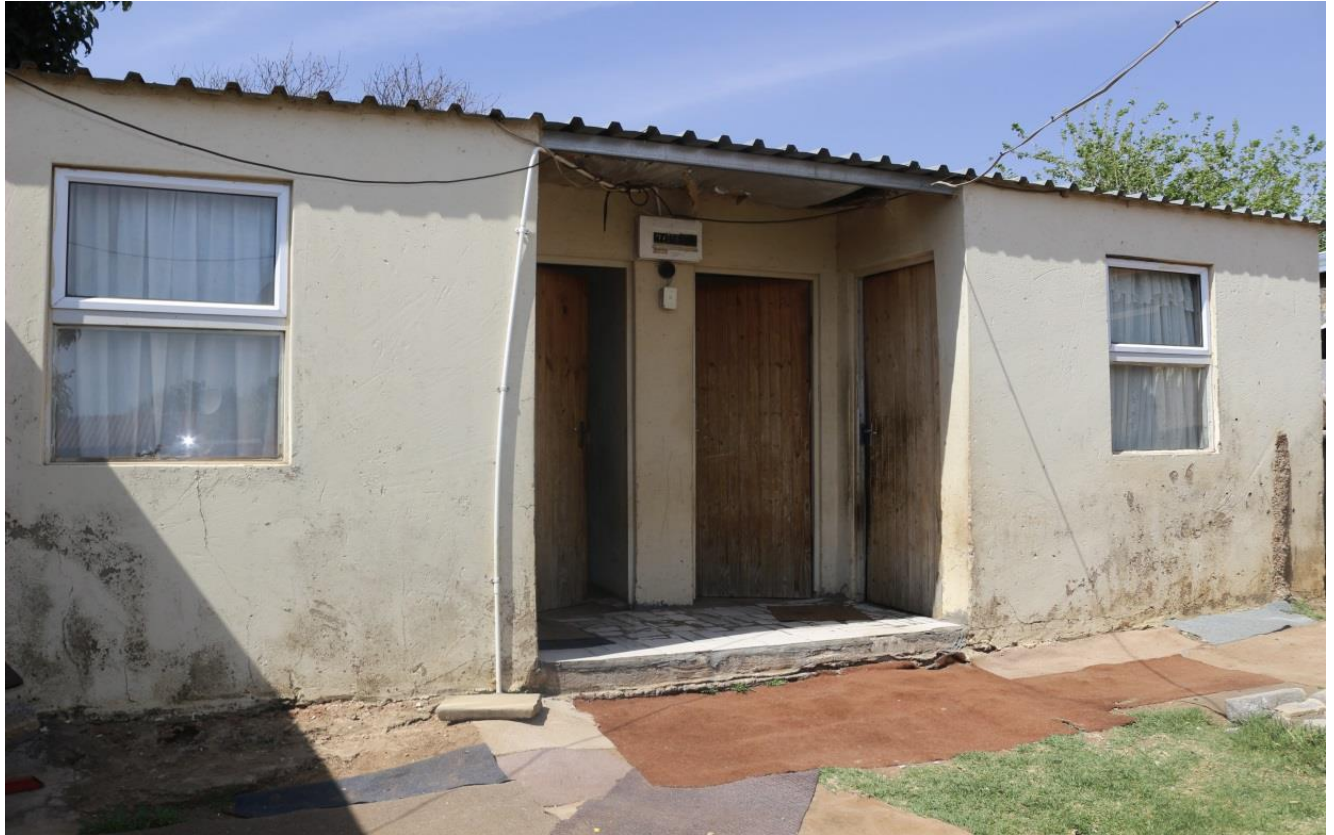
Upgraded units in the backyard of old council housing in Zola ©Hopa, 2016
