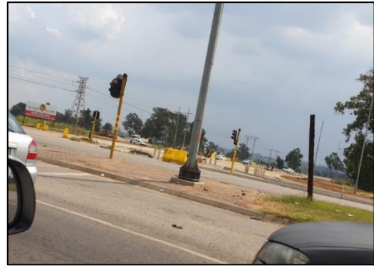
Figure 18: Rondebult road and Espri Avenue intersection road extension construction by south entrance of Checkers Hypermarket.
