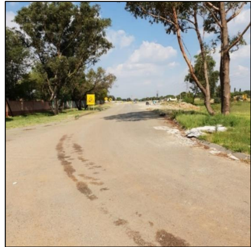
Figure 19: Rondebult road and Espri Avenue intersection road extension construction by south entrance of Checkers Hypermarket.
