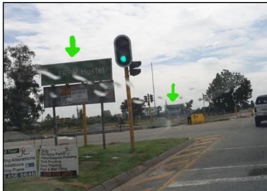
Figure 17: Rondebult road and Espri Avenue intersection road extension construction by south entrance of Checkers Hypermarket (marked with green arrows).
