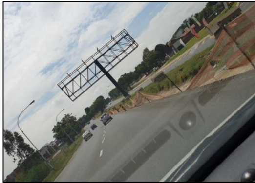
Figure 16: Rondebult Avenue road construction (width) south bound across from the Urbika Lifestyle Estate (south of Parkdene phase of Leeuwpoort).
