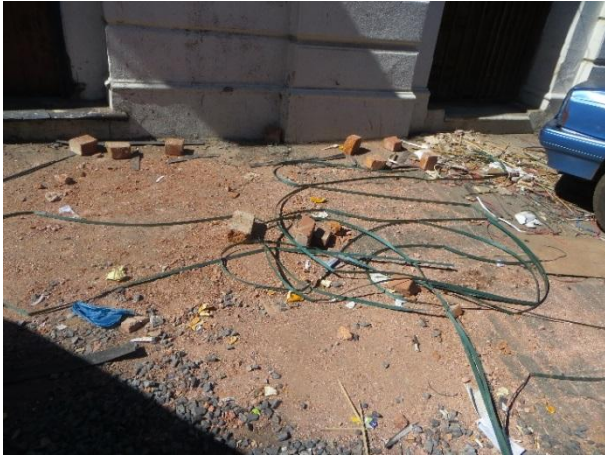
Photo 4.24 Poor pedestrian environments just outside of the Precinct off Commissioner Road.
