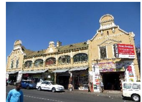
Photo 6.12 Different building typologies for preservation and interesting meaningful architecture and spaces.
