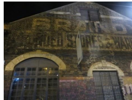
Photo 4.3. Preservation of historic buildings now converted to Arts on Main.
