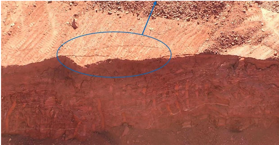
Figure 4.8: Cracks forming on the crest of an open pit highwall (Thomas, 2020)
