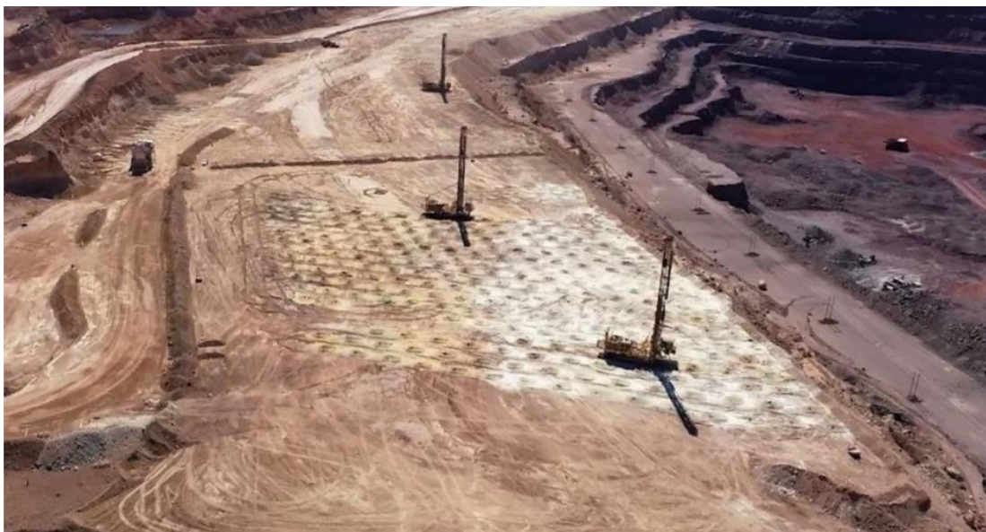
Figure 4.9: An aerial view of a designed blast pattern being drilled (Thomas, 2020)
