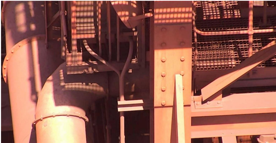
Figure 4.6: A closer aerial inspection of the bolts and fittings of a processing plant (Thomas, 2020)
