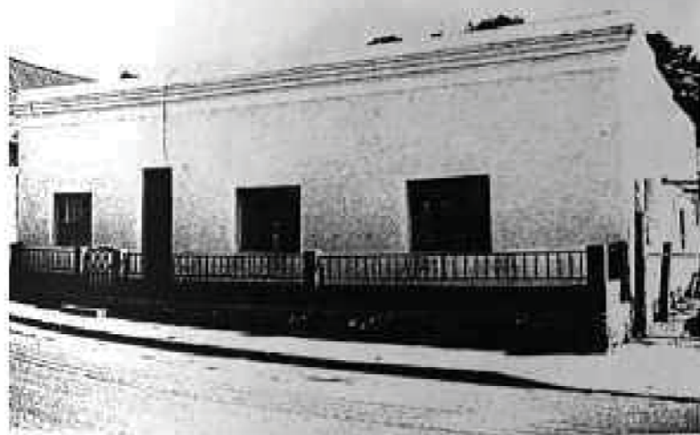
Erven 380 & 381: 26 Stockenstrom Street.
