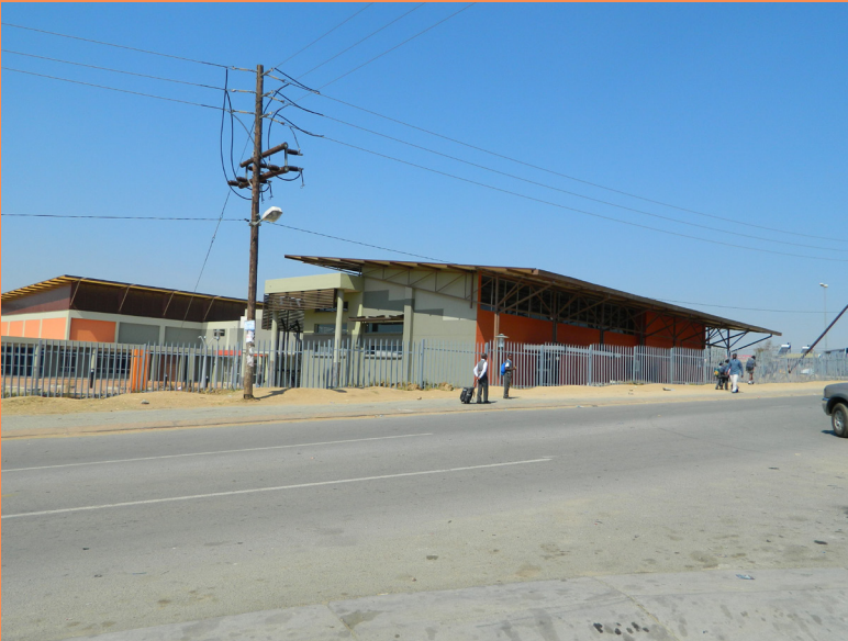
Cosmo Community Centre: The building is fenced off and does not respond to the street edge
