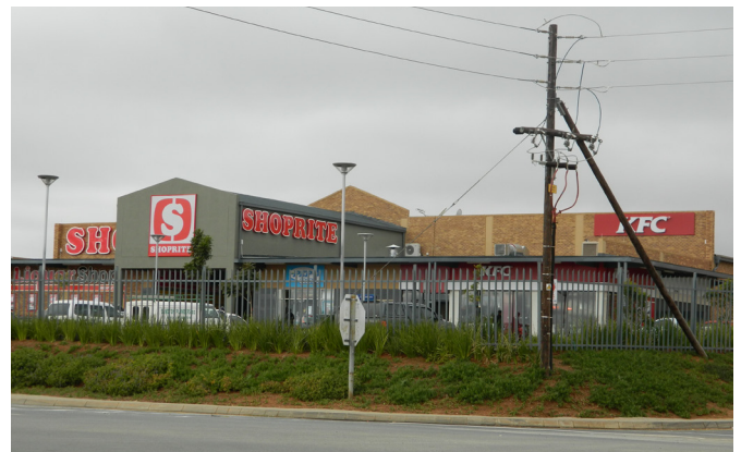
Shopping centre located along the Corner of South Africa Drive and Malibongwe Drive
