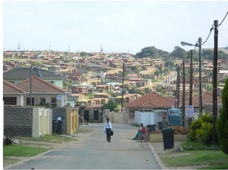
The chaotic mix of housing typologies: The image shows the bonded houses in the foreground, with an endless view of the low cost houses in the background
