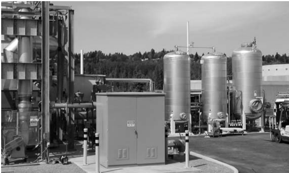
Figure31: A Suburban Scale Bio-gas Application: The world's largest fuel cell demonstration project under way in a Seattle suburb
