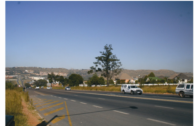
1: View down Christiaan De Wet. (lack of street lighting)
