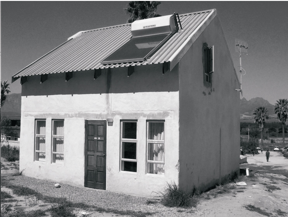
A Double Storey Houses in the Scheme built with ecobond bricks
