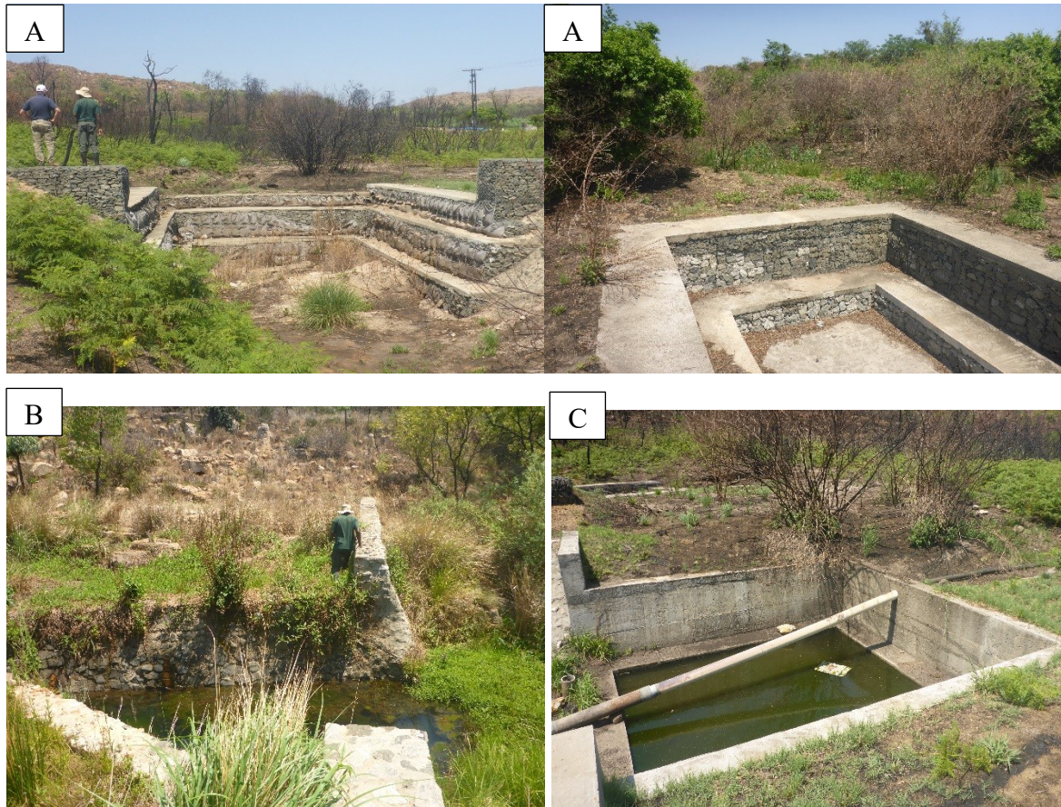
Figure 11: Erosion control and stabilisation interventions recorded on a wetland on site. (A) – gabion concrete cast weirs, (B) – rock masonry and (C) – concrete drop inlet weir.
