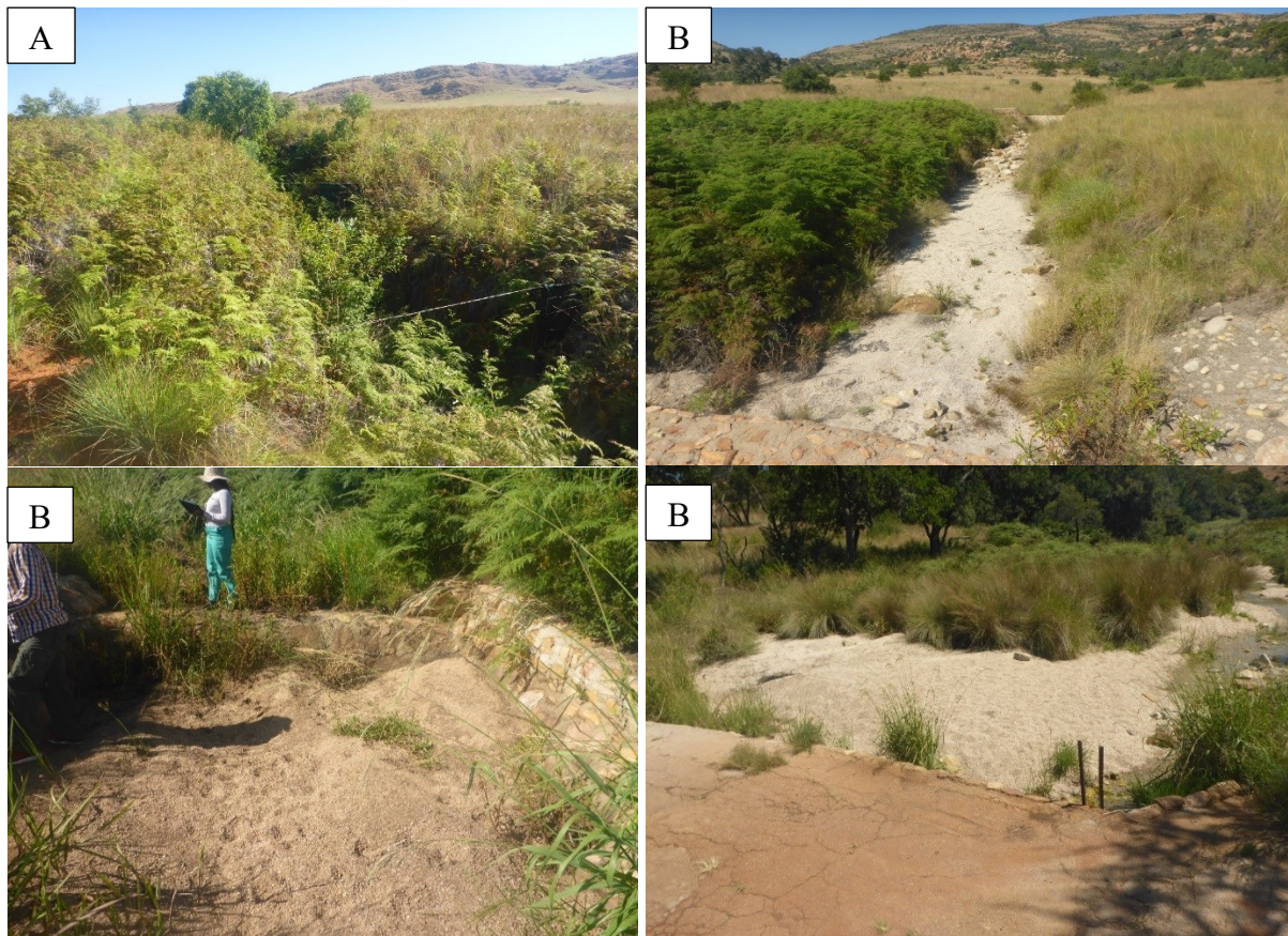
Figure 8: Channel incision and sediment fences (A) within side slopes of UCVB1, exposed sediment bars upstream and downstream of the flow impeding structures (B) within CVB1 within the Kgaswane Nature Reserve.
